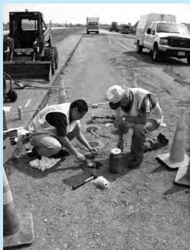
A strain gage is installed at the MnROAD facility.
