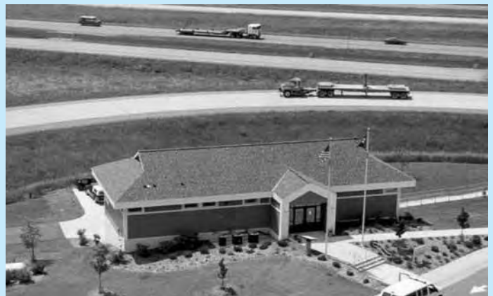
MnROAD building, with a five-axle trailer passing on the Low-Volume Roadway immediately behind, and Interstate 94 and the High-Volume Roadway in the background.
