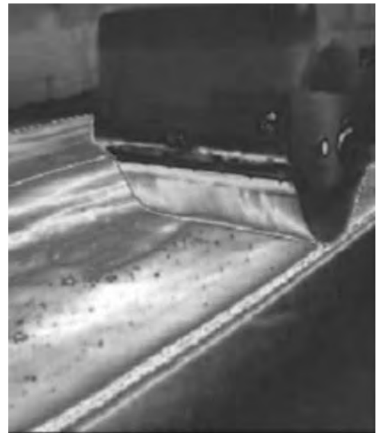
Infrared imagery was used to study techniques for the application of hot-mix asphalt.
