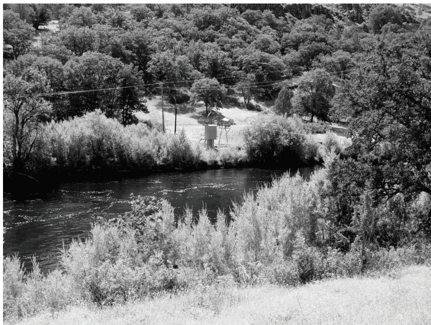
FIGURE 4-2 The U.S. Geological Survey stream gauge site on the Klamath River immediately below Iron Gate Dam is the site for calculated natural flows and recommended instream flows. The gauge site includes a cable car for sampling and a rectangular housing for data recorder and transmitter.
