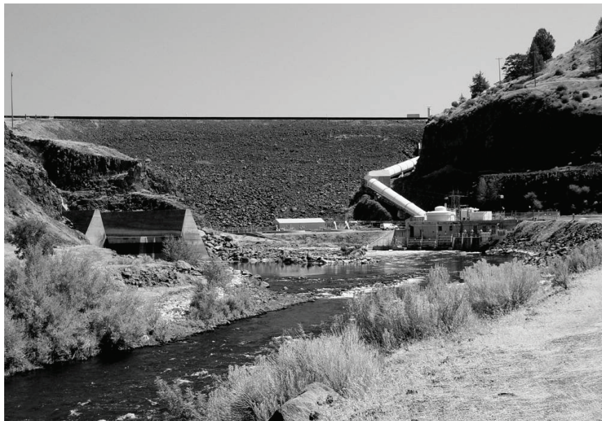
FIGURE 1-2 Iron Gate Dam on the Klamath River is the dividing point between the upper and lower Klamath River basins. The penstock for the power generators is on the right, and the spillway is on the left in this view looking upstream.
