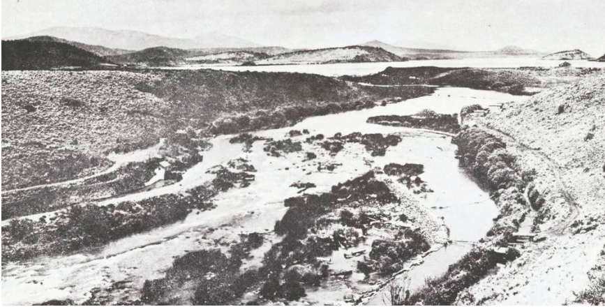
FIGURE 2-2a This reach of the Link River below Upper Klamath Lake, shown here in 1919, is the site of Link River Dam. Note the bedrock outcrops forming ledges and rapids in the channel that act as a sill for the level of the lake upstream. SOURCE: Boyle 1976. Reprinted with permission; copyright 1976, Klamath County Museum.
