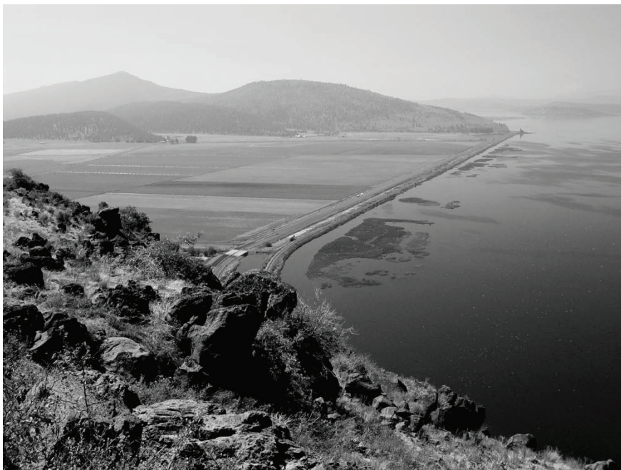
FIGURE 4-6 The NFS adjusted flows from the upper Klamath River basin to account for the conversion of marsh areas to agriculture, such as shown here on the southeast side of Upper Klamath Lake. Levees separated the area now under cultivation (on the left) from the lake and its marsh area (on the right).
