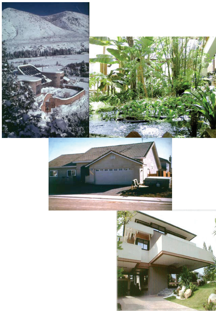
FIGURE 10.2 Top : Amory Lovins' house (and the original headquarters of the Rocky Mountain Institute) in chilly Snowmass, Colorado ( left ), uses about 1 percent the normal space- and water-heating energy and 10 percent the normal electricity, with a 10-month payback in 1983. It has produced 28 indoor banana crops ( right ) with no furnace. Middle : A Davis, California, tract house, designed by Davis Energy Group to use about a tenth the normal U.S. amount of energy, is comfortable with no air conditioner at up to 115°F (45°C) and, if built in quantity, would cost about $1,800 less than normal to construct and $1,600 less over time to maintain. Bottom : Designed and constructed by Professor Dr. Soontorn Boonyatikarn, this 350-square-meter Bangkok house, at normal construction cost, provides superior comfort with one-tenth the normal air-conditioning energy. SOURCE: Top : Courtesy of Rocky Mountain Institute. Bottom : Courtesy of Soontorn Boonyatikarn, Chulalongkorn University.
