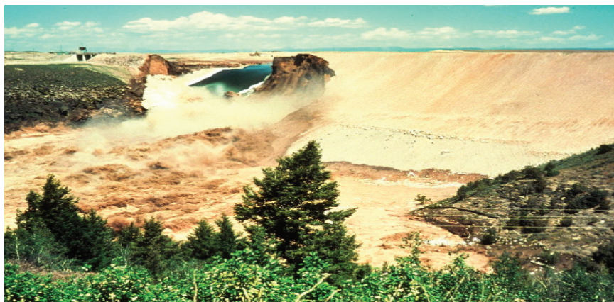
FIGURE 1.2 Teton Dam failure. View northwest toward the breach. The canyon floor is flooded from bank to bank, and all works there are completely inundated. SOURCE: BOR.
