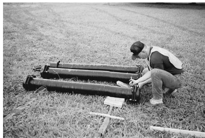
Figure 4.8. Ductile iron pipes wired and capped.
