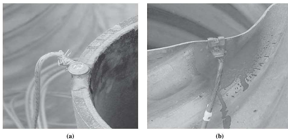
Figure 4.23. Wiring of ductile iron pipes and corrugated steel culverts.
