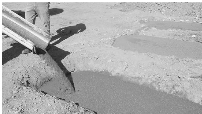
Figure 4.11. Backfilling trenches with CLSM.
