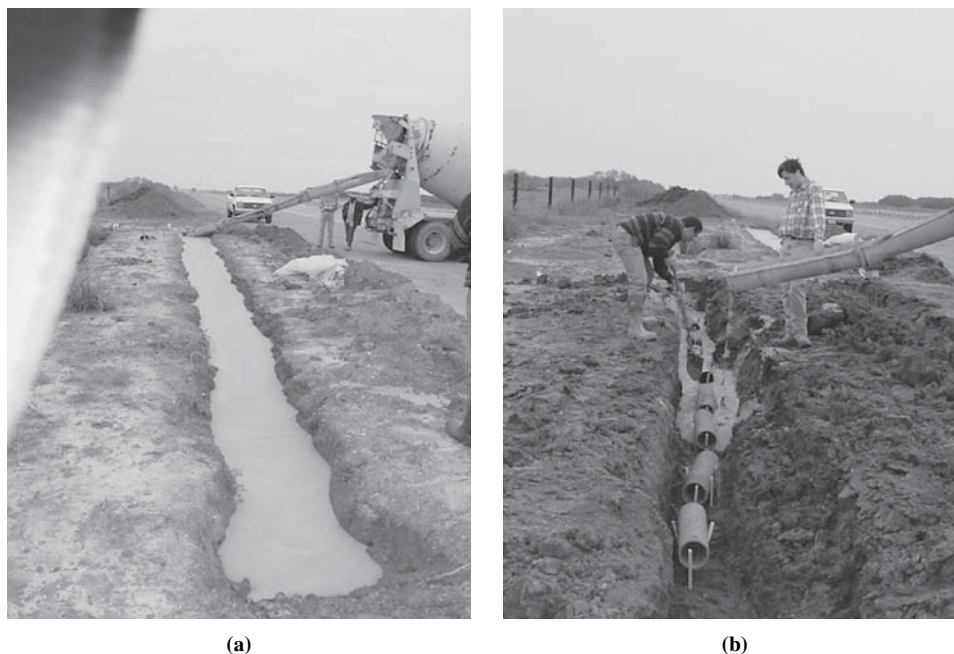
Figure 4.26. Placement of CLSM into the trenches.
