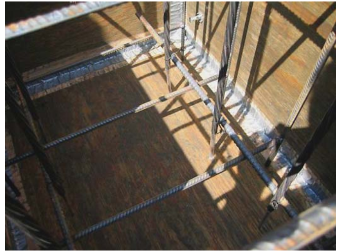
Figure B-23. View of inside of form.
