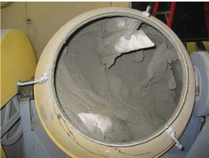
Figure B-34. Mortar in mixer.
