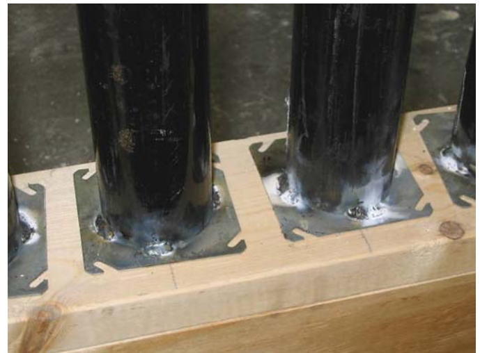
Figure B-43. End plates welded to pipe bases.
