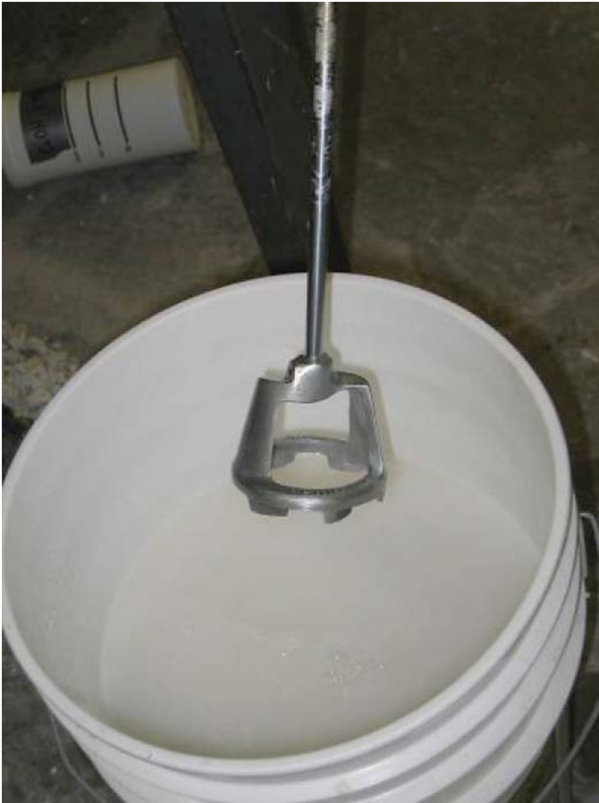
Figure B-44. Mixture in bucket and mixing attachment to drill.
