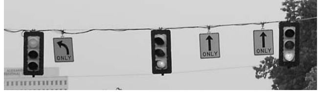
FIGURE 12 MUTCD overhead lane-use control signs.
