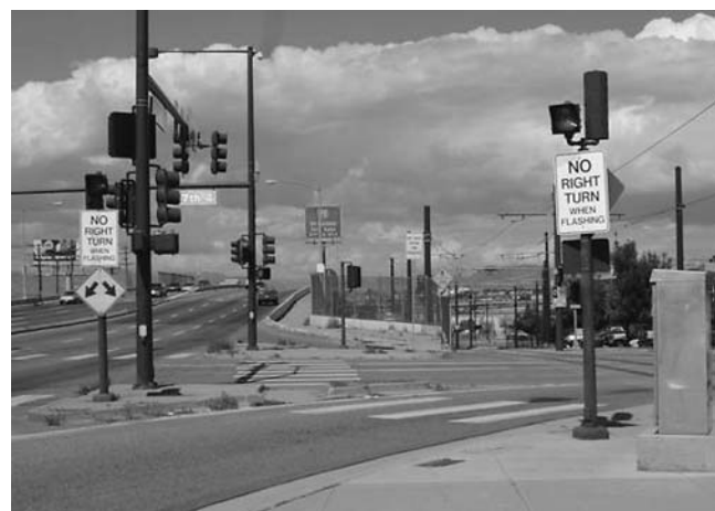
FIGURE 28 No Right Turn When Flashing sign from Colfax Avenue to 7th Street in Denver.
