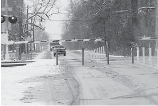
FIGURE 2 Retractable barriers under test in Wayne County, Michigan (Courtesy: Michigan Department of Transportation).
