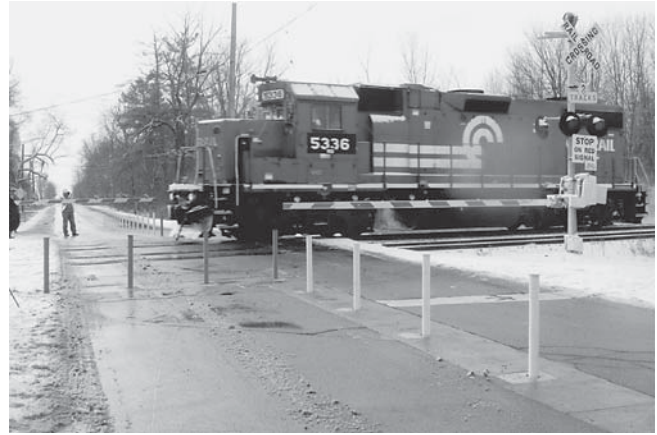
FIGURE 2 Retractable barriers under test in Wayne County, Michigan (Courtesy: Michigan Department of Transportation).
