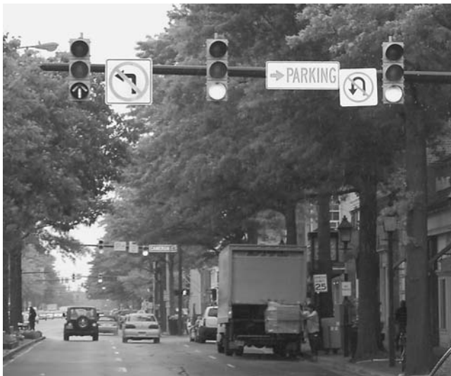
FIGURE 15 Example of sign clutter and misplacement.
