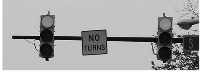
FIGURE 16 Use of the MUTCD No Turns sign.
