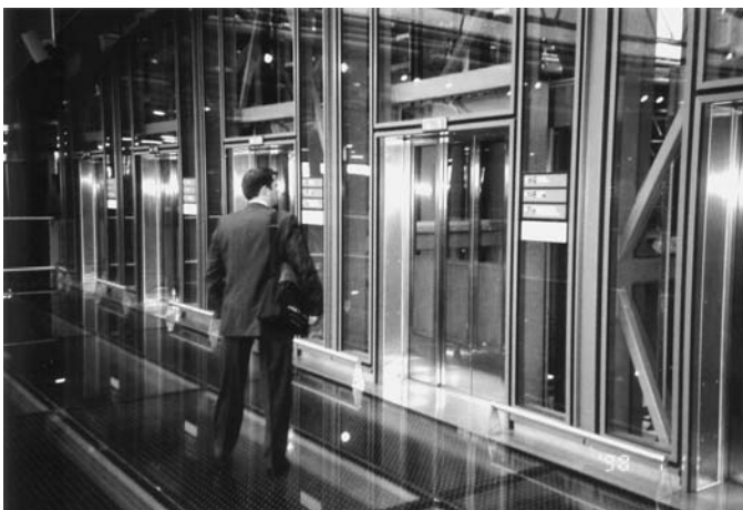
Figure 4-15. Heathrow Airport Terminal 5—high-capacity flow-through elevators. Source: Corgan Associates, Inc.
