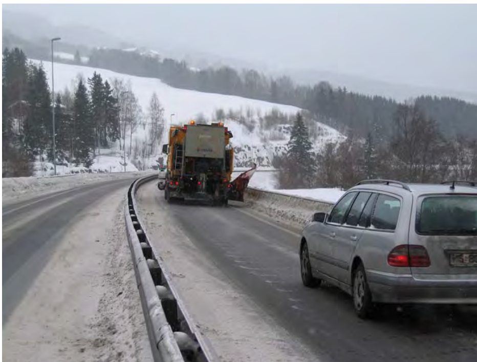
FIGURE 2 Two-lane road with crash barriers on central reserve.
