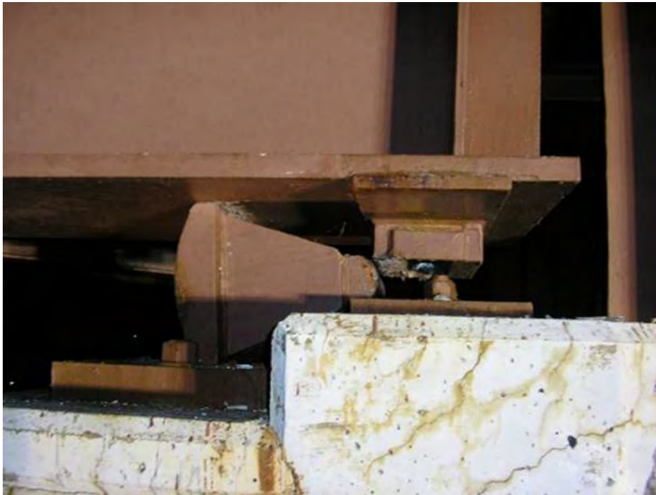
FIGURE 3 Earthquake-type damage.
