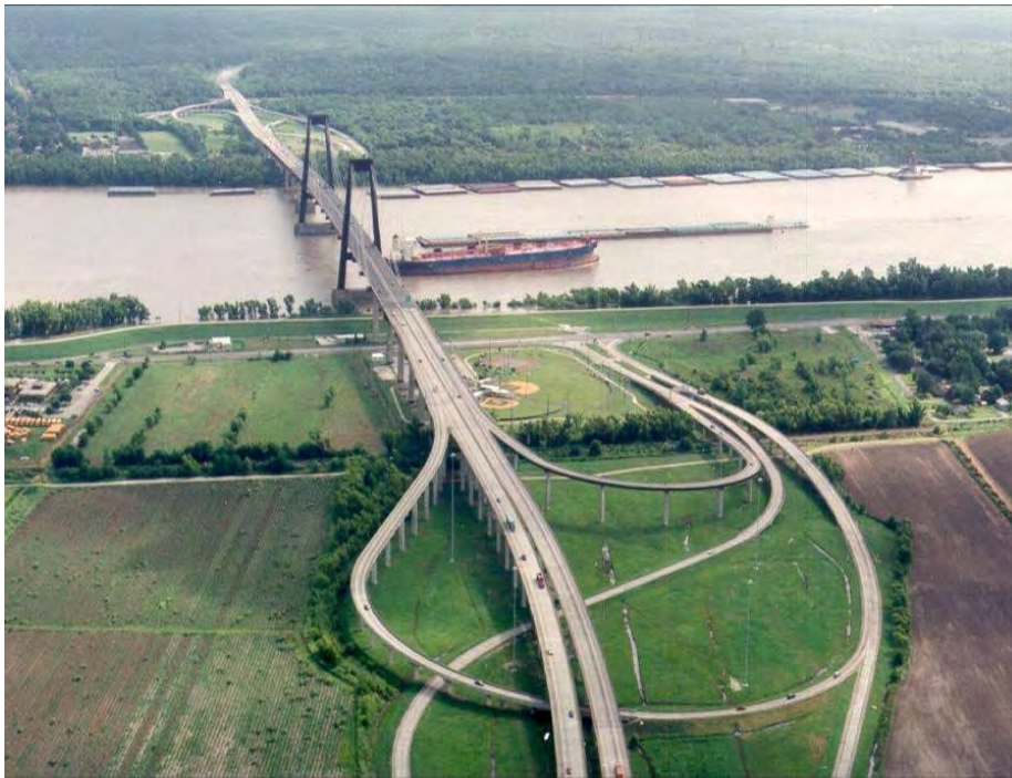
FIGURE 1 Hale Boggs Memorial Bridge alignment [Louisiana Department of Transportation Development (LaDOTD) photo].
