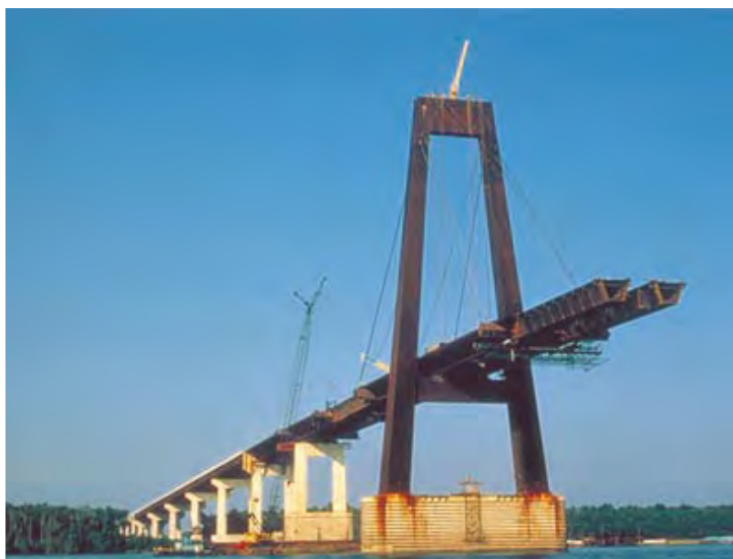
FIGURE 3 Hale Boggs Bridge under construction (LaDOTD photo).
