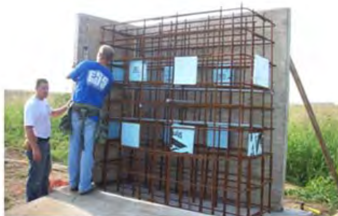
FIGURE 1 Photograph of test block during construction.
