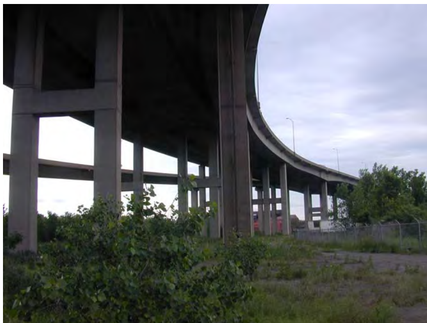
FIGURE 1 A view of the cast-in-place box girder bridge.
