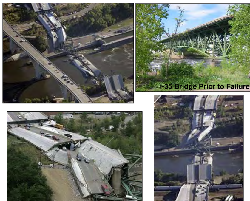
FIGURE 7 Collapse of the I-35 bridge in Minneapolis, Minnesota.
