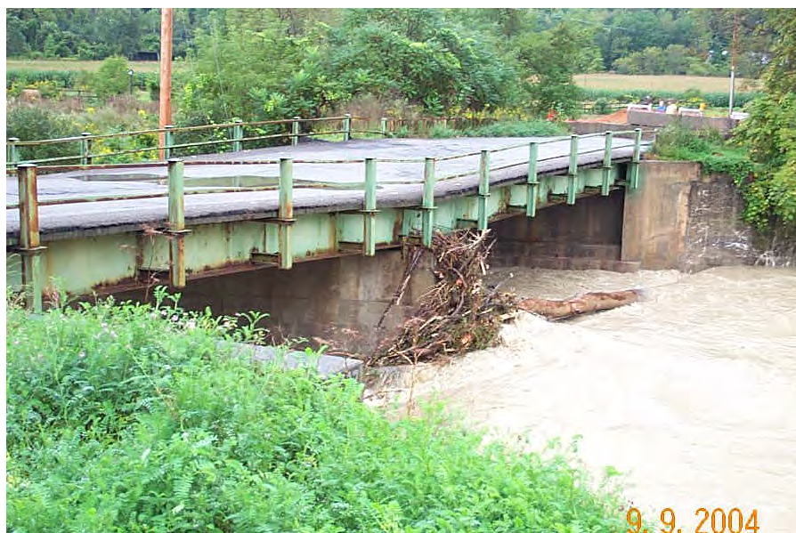
FIGURE 4 Scour damage.
