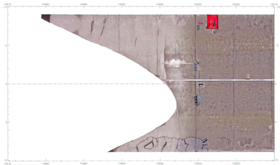
FIGURE 10 Tunnel inspection photo.
