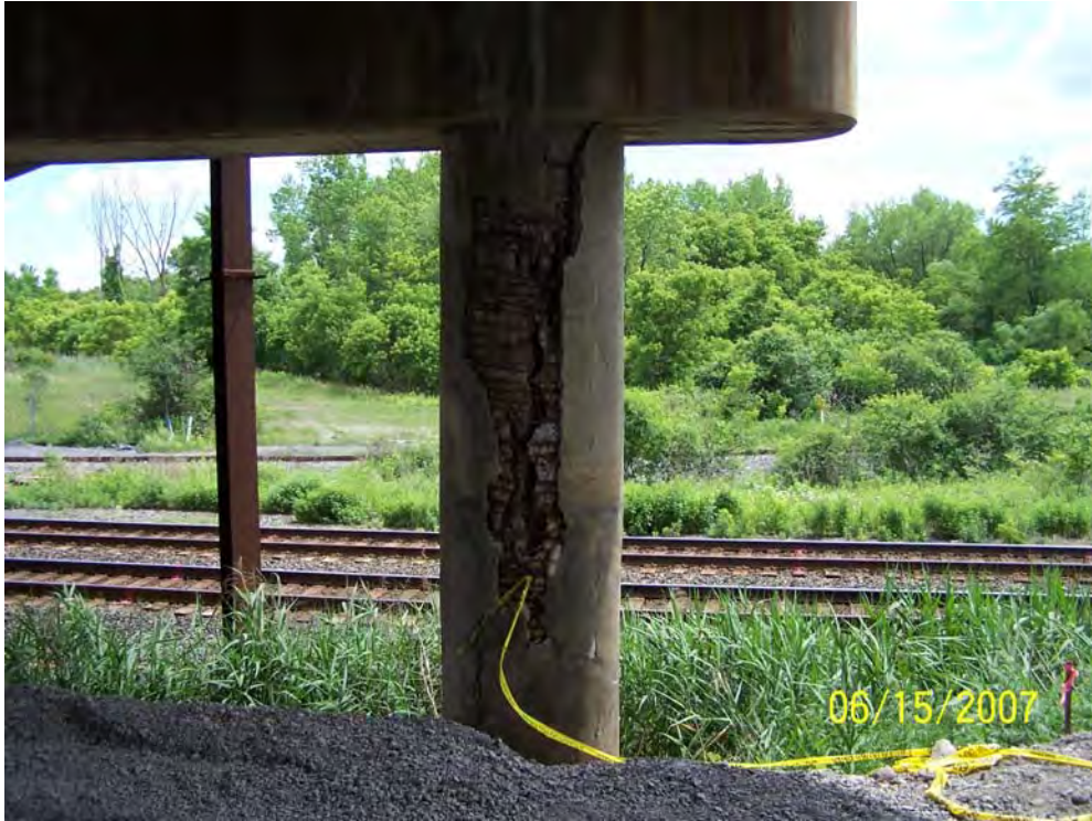
FIGURE 2 Corrosion damage.
