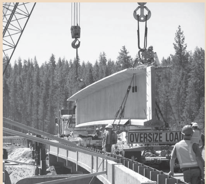
Bridge program contractors install one of seven record-breaking precast concrete beams—manufactured in-state—at the Union Pacific Railroad overcrossing near Chemult, Oregon.
