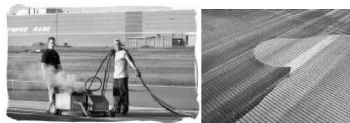
FIGURE C17 Sand blasting unit and runway rubber removal results.
