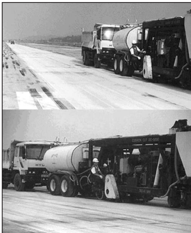
FIGURE C15 Diamond grinder in operation on airport (McLake 1999).
