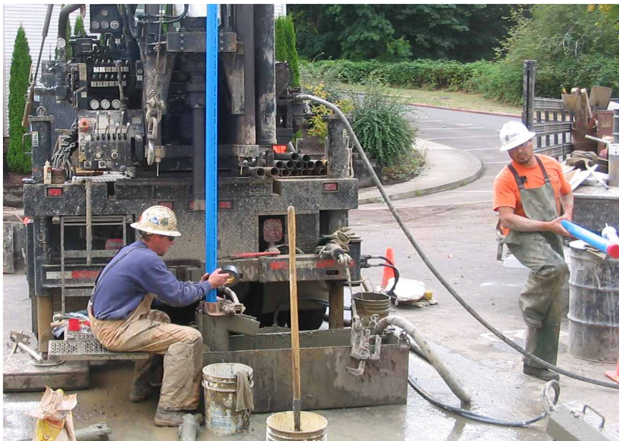
FIGURE 10 Installation of inclinometer casing in a vertical borehole (Landslide Technology).
