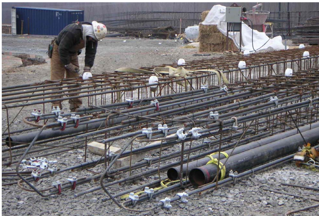
FIGURE 14 Eight-inch steel pipe placed within diaphragm wall reinforcement for housing inclinometer casing (Case Foundation Co.).
