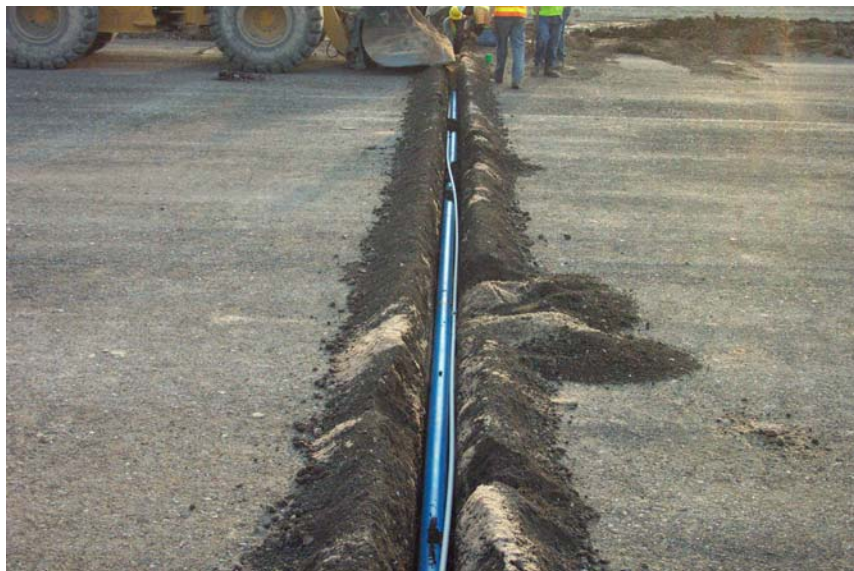
Inclinometer installed for monitoring settlement of base (Puppala).
