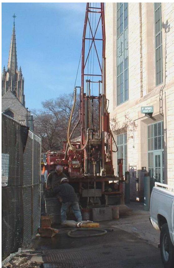
Inclinometer installed between a shored excavation and an existing building (Blackburn).
