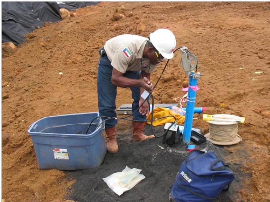
FIGURE 18 Performing measurements using a traversing inclinometer probe and data recording device (Landslide Technology).
