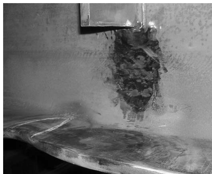
Figure 2.23. Completed heat-straightening repair at stiffener detail.
