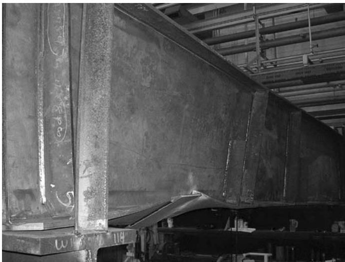
Figure 1.23. Before and after a heat-straightening repair.
