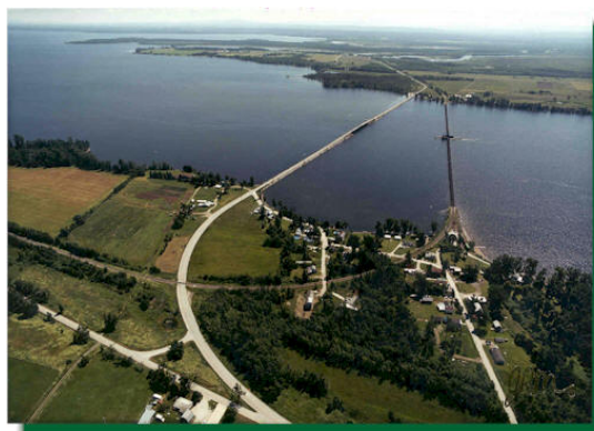
FIGURE 7 Missisquoi Bridge over Lake Champlain.
