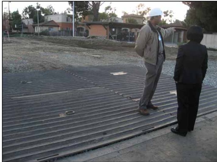
FIGURE 5-10 Rumble strips to remove dirt from vehicle tires. SOURCE: Laura Ehlers, National Research Council.
