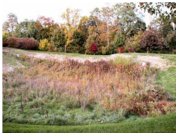
FIGURE 5-43 Dry extended detention pond. SOURCE: PaDEP (2006).
