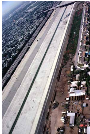
FIGURE 3-25 Example of a channelized urban stream for maximized flood conveyance and geomorphic stability (Los Angeles River, California). SOURCE: Robert Pitt, University of Alabama.
