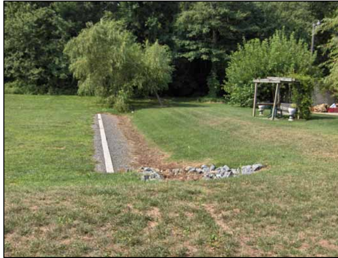
FIGURE 5-11 Level spreader. SOURCE: Robert Traver, Villanova University.
