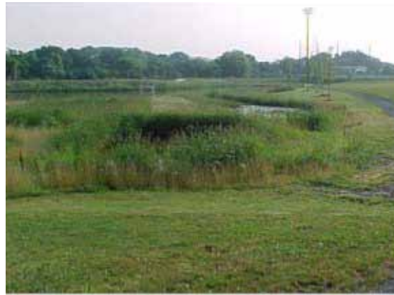
FIGURE 5-40 Constructed wetland. SOURCE: PaDEP (2006).
