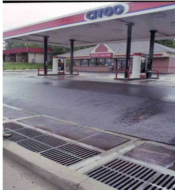
FIGURE 5-46 Delaware sand filter. SOURCE: Tom Schueler, Chesapeake Stormwater Network.
