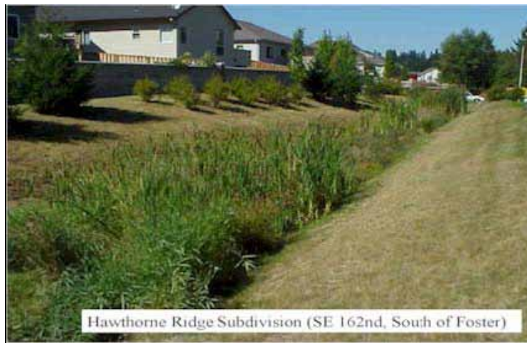
FIGURE 5-16 Vegetated swale. SOURCE: PaDEP (2006).
