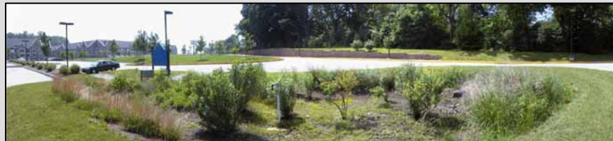
FIGURE 5-21 Villanova Bioinfiltration Traffic Island SCM. SOURCE: Reprinted, with permission, from VUSP. Copyright by Villanova Urban Stormwater Partnership.
