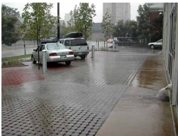
FIGURE 5-32 A small office building conversion at the edge of downtown Denver included the replacement of a portion of the site's parking with modular block porous pavement underlain by an 18-inch layer of crushed rock. Rainfall on the porous pavement and roof runoff for most storm events are contained in the reservoir created by the crushed rock. The pavement infiltrates runoff from most storm events for one-third of the impervious area on the half-acre site. SOURCE: Courtesy of Wenk Associates.
