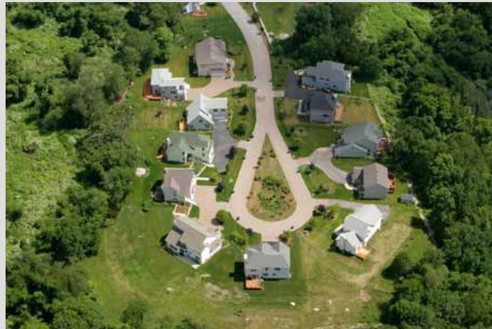
FIGURE 5-37 Jordan Cove LID subdivision. SOURCE: Reprinted, with permission, from Clausen (2007). Copyright 2007 by John Clausen.
