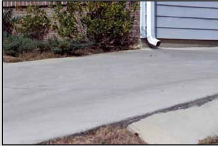
A directly connected roof drain
