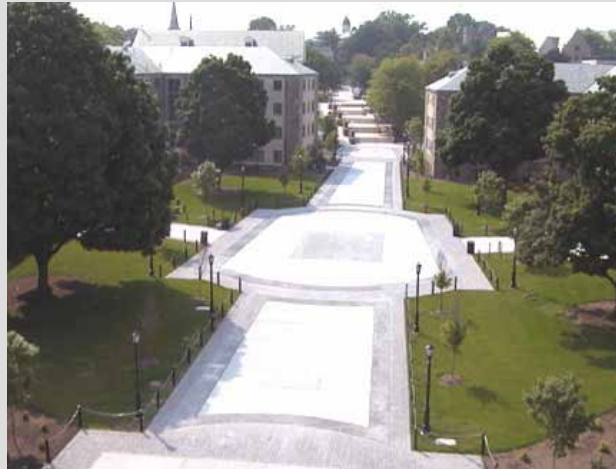
FIGURE 5-33 Villanova University pervious concrete retrofit site. SOURCE: Reprinted, with permission, from VUSP. Copyright by VUSP.
