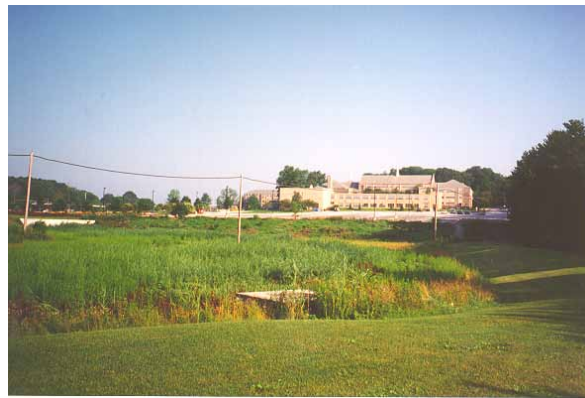
FIGURE 5-41 Retrofitted stormwater wetland at Villanova University. SOURCE: Reprinted, with permission, from VUSP. Copyright by VUSP.
