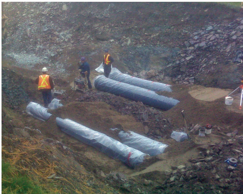
FIGURE 3-1 Example of ductile iron pipe encased in polyethylene. SOURCE: Courtesy of Daniel Crabtree, Ductile Iron Pipe Research Association.
