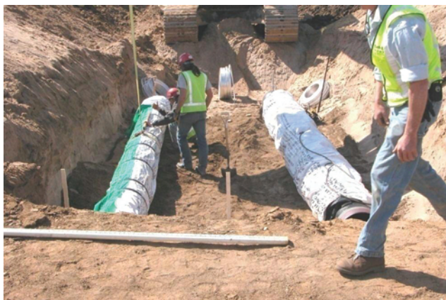
FIGURE 3-6 Ductile iron pipe with polyethylene encasement and a ribbon galvanic anode cathodic protection system. SOURCE: Courtesy of William Spickelmire, RUSTNOT Corrosion Control Services, Inc.
