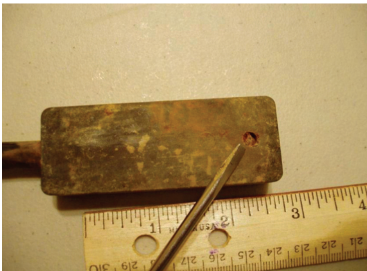
FIGURE D-5 From Mid-Dakota Rural Water Service Project, South Dakota: failed Probe No. 3, following removal, showing manufacturing defect. SOURCE: Courtesy of Schiff Associates, Claremont, California.
