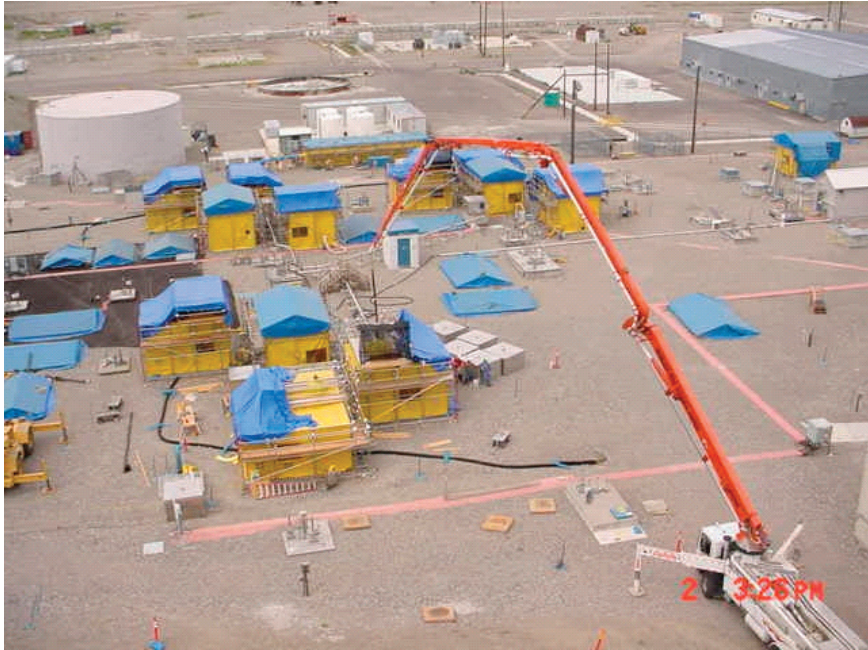
FIGURE 2.8 Tremie being used to emplace grout in a tank at the INL site. The use of tremies (long flexible pipes) is common in the construction industry. For EM's applications, the components of specially formulated grout mixtures must not separate before they reach their in-tank destination and solidify. SOURCE: Department of Energy.
