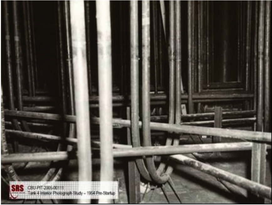
FIGURE 2.3 Cooling coils in an SRS tank. Such coils maintained the temperature of high-level radioactive waste below boiling. The coils are an obstacle to removing the tank waste at SRS.
