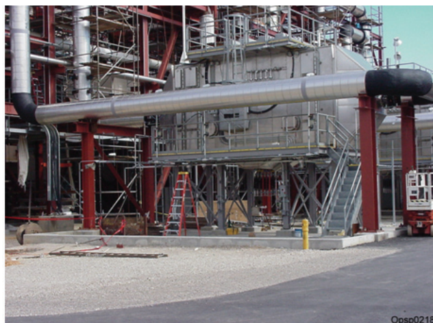
FIGURE 2-5 PFS filter unit. SOURCE: Robie Jackson, Waste Management Manager, ANCDF, and Tracy Smith, Trial Burn Manager, ANCDF, "The use of carbon at ANCDF," Presentation to the committee, June 5, 2008.
