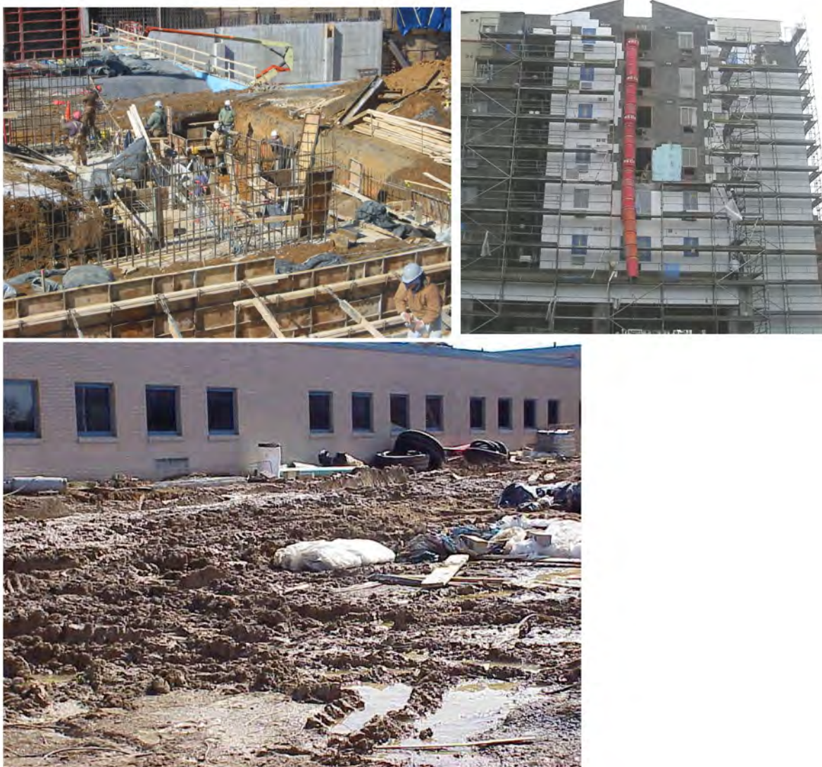
FIGURE 1.1 Examples of on-site construction methods and weather issues. SOURCE: Thomas (2008).
