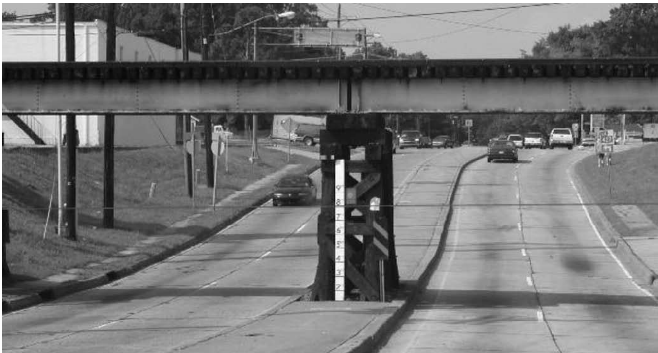
FIGURE 9 Passive underpass flood depth gauge (Baton Rouge, Louisiana). (Note: the horizontal line indicates the 8-ft flood depth during Tropical Storm Allison in 2001.)
