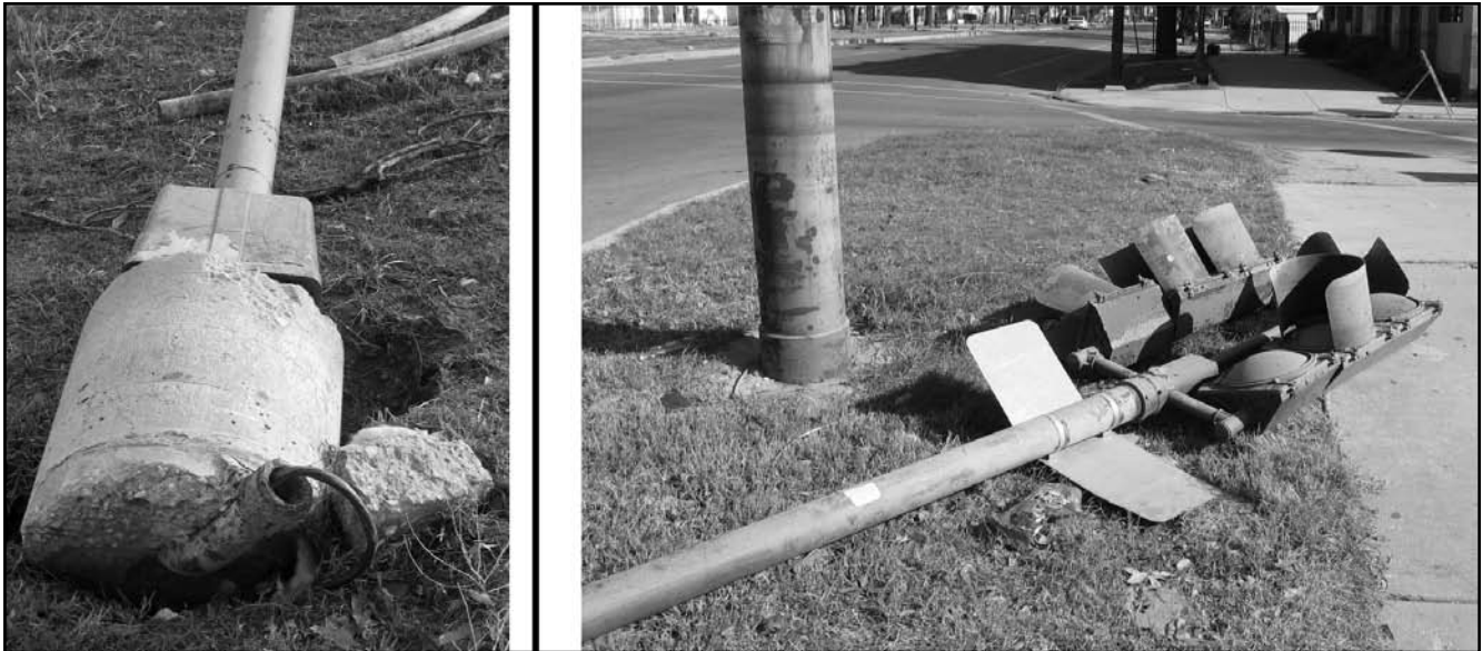
FIGURE 20 Foundation damage to pedestal mounted signal (Dykes 2006).
