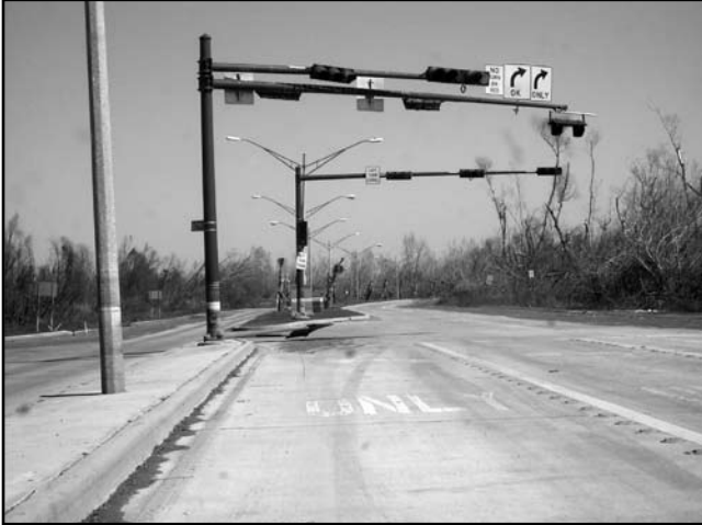
FIGURE 19 Wind and flood damage to mast arm signal location (Dykes 2006).
