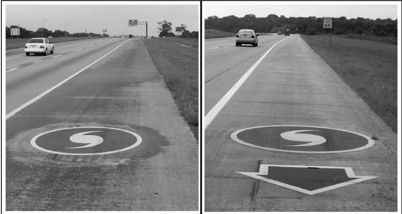
FIGURE 10 Hurricane evacuation route directional shoulder pavement markings (normal lanes at left and contraflow lanes at right), US-290, Texas. (Note: photos not taken under evacuation conditions.)
