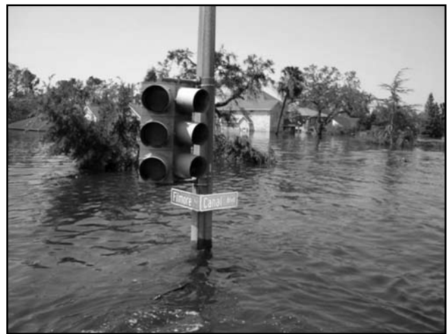
FIGURE 18 Flooded signalized intersection in New Orleans (Dykes 2006).
