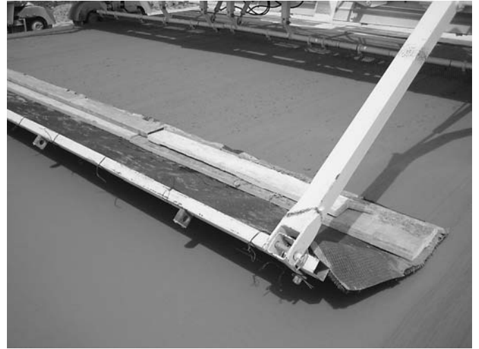
Figure 4-6. Heavy turf drag texturing.
