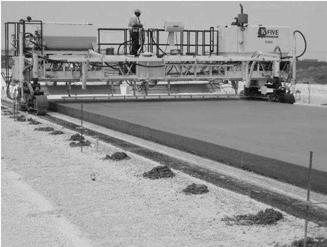
Figure 4-4. Longitudinal tining.
