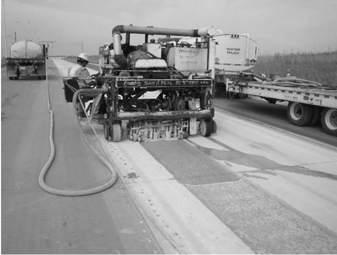
Figure 4-15. Longitudinal grooving machine.
