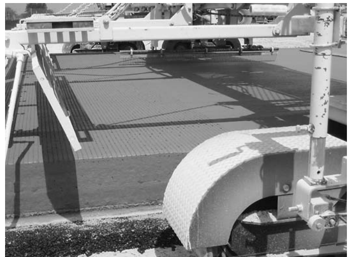
Figure 4-8. 0.5-in (12.7-mm) transverse tining (Section 9).
