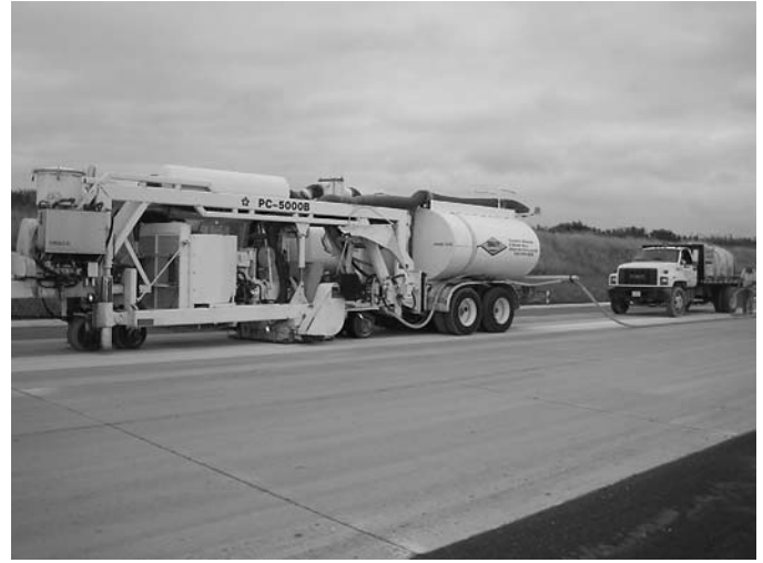
Figure 4-12. Diamond grinding machine.
