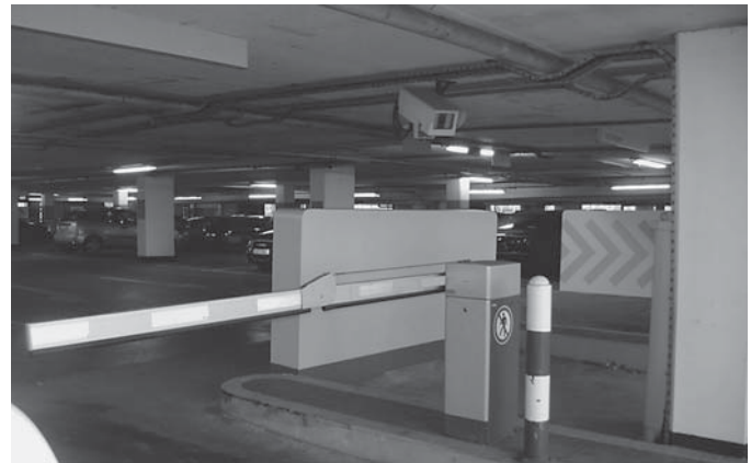
Figure E.6a. Entry gate and license plate recognition camera at Dublin Airport.
