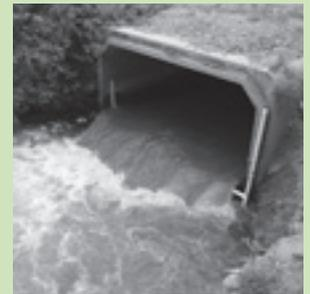
*A concrete box culvert in a medium- to high-gradient mountain stream. The culvert width is less than the width of the stream channel; therefore, during high flows, as shown in the photo, the constriction creates a velocity barrier to the upstream passage of most fish species. Because the water velocities also create scouring downstream, the culvert includes an outlet drop, which fish must negotiate in addition to the water velocities within the structure.*
