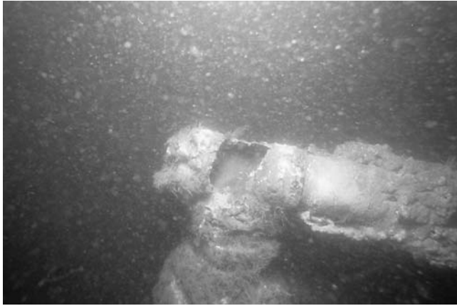
FIGURE 24 Underwater sonar bracket installation in the tidal environment showing corrosion.
