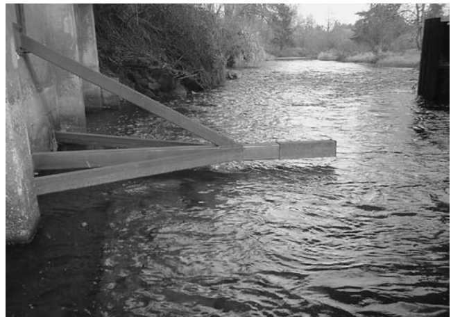
FIGURE 49 Close-up of a sonar scour monitor on the Kline Bridge.
