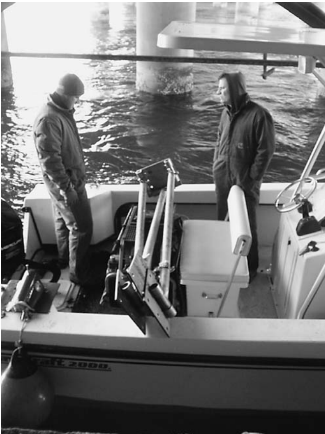
FIGURE 27 Installation of an underwater sonar bracket requires divers and a boat.
