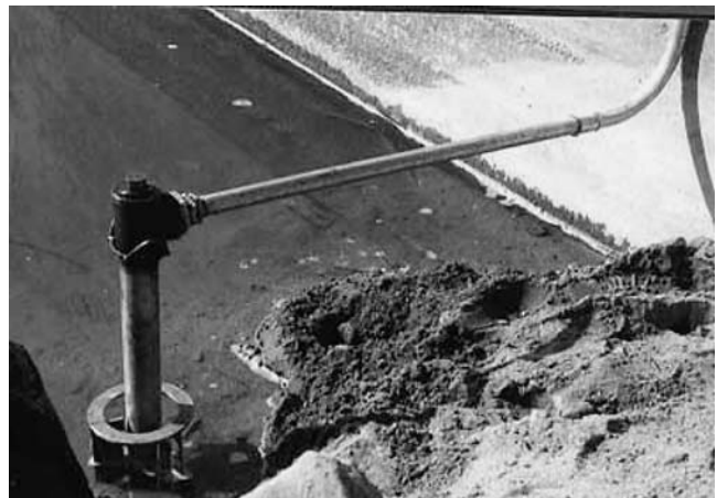
FIGURE 8 Magnetic sliding collar installation.
