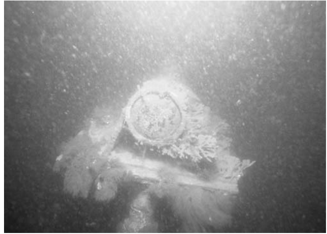
FIGURE F7 Marine growth on a sonar scour monitor.
