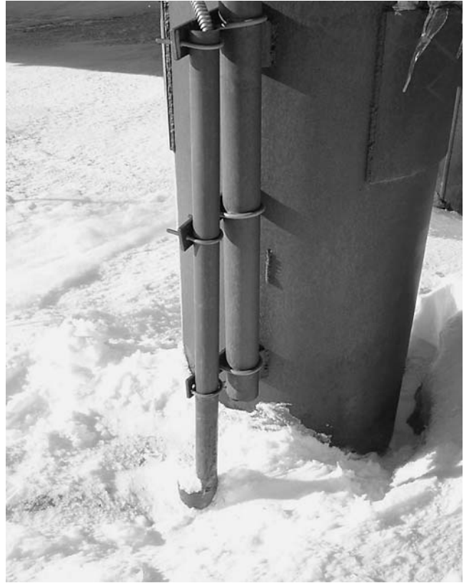
FIGURE 22 Sonar monitor mounted on pier in the snow in Alaska.
