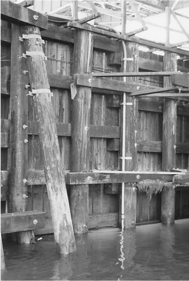
FIGURE 30 Close up of velocity meter mounted on the fender of the Woodrow Wilson Bridge.
