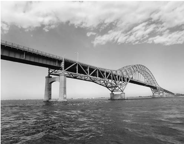
FIGURE 42 Elevation of Robert Moses Causeway over Fire Island Inlet, Long Island (Copyright: Raimondo di Egidio).
