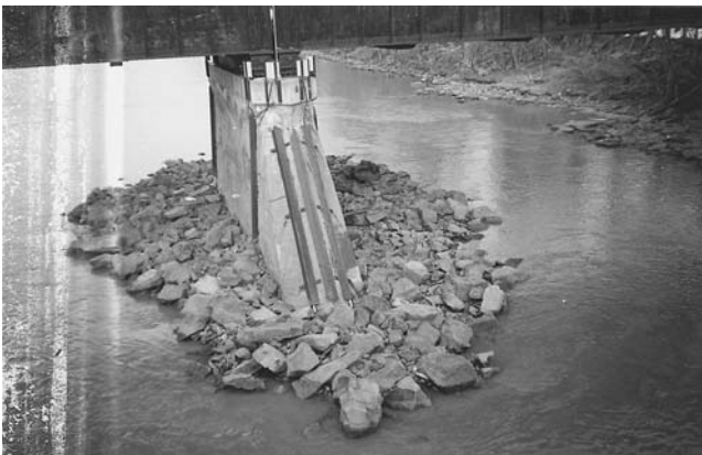
FIGURE 14 Sounding rods installed to monitor riprap in New York.
