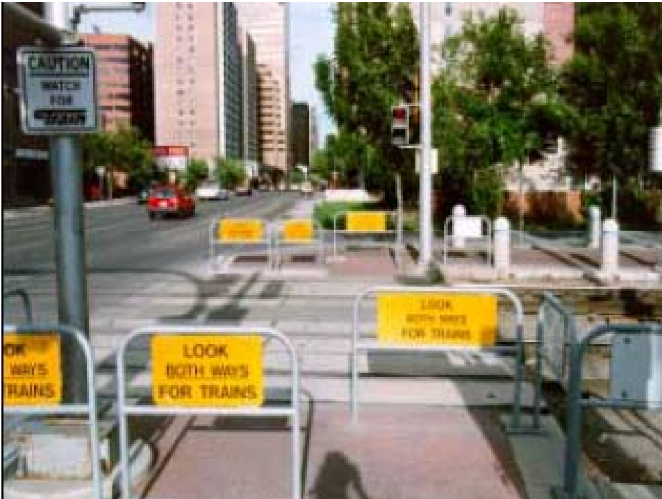
Figure 10: Example of bedstead crossing (Calgary, Alberta)
