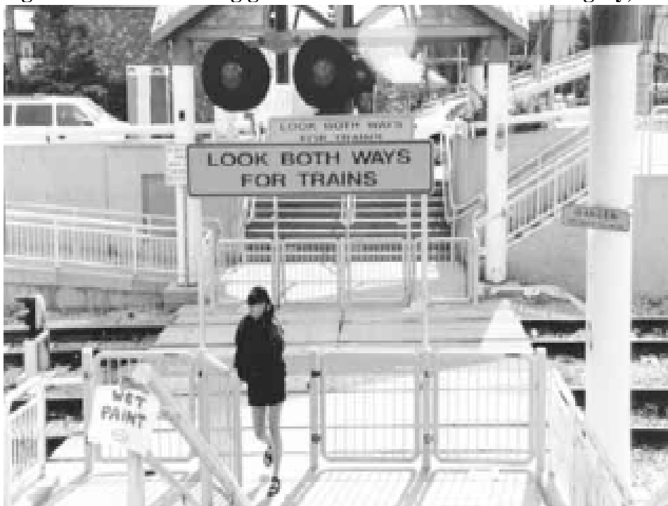
Figure 18: Manual swing gates with overhead flashers in Calgary, Alberta
