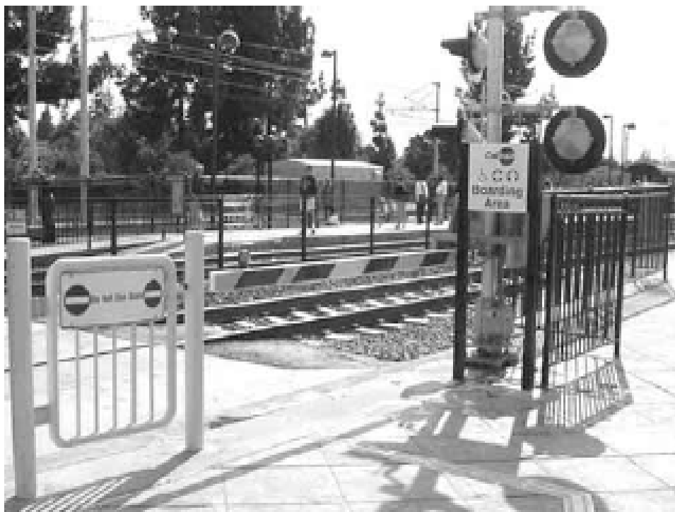
Figure 17: Pedestrian automatic gates and swing gates
