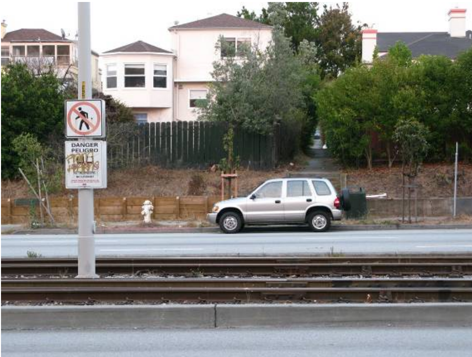
Exhibit 26: Break in Intertrack Fencing Opposite Community Access
