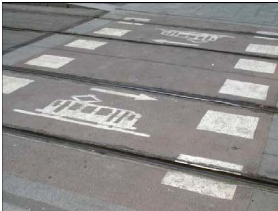
Figure 6: LRV directional striping (one-way track) in Barcelona, Spain
