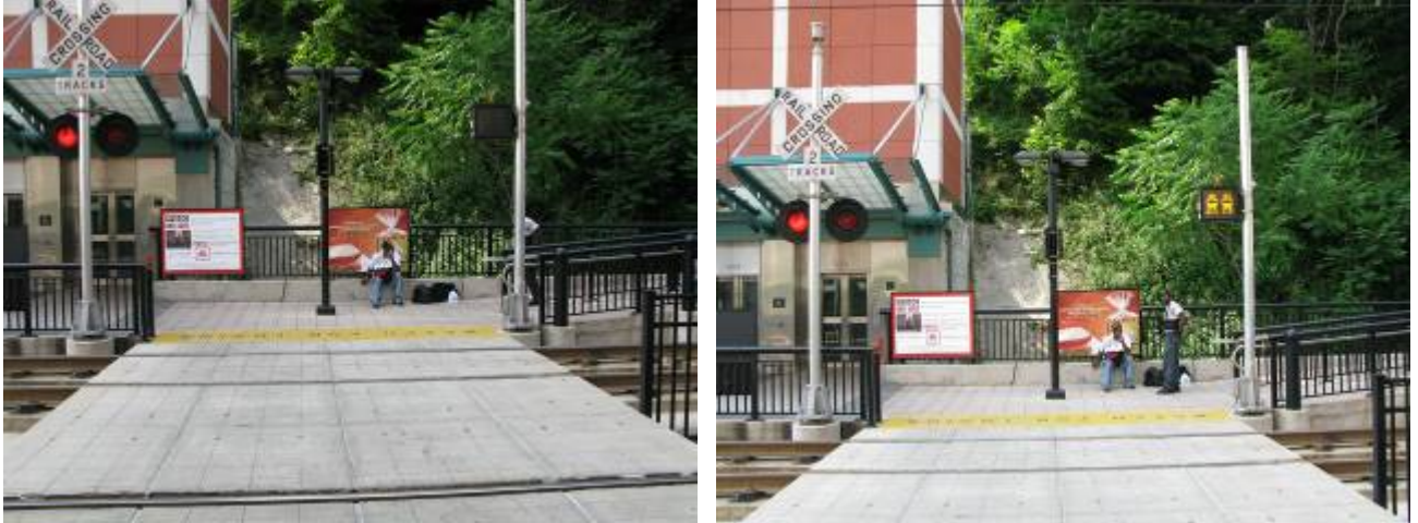
Exhibit 4: Second Train Coming Blank Out Sign at Pedestrian Crossing (Left: Before First Train, Right: Between First and Second Trains)
