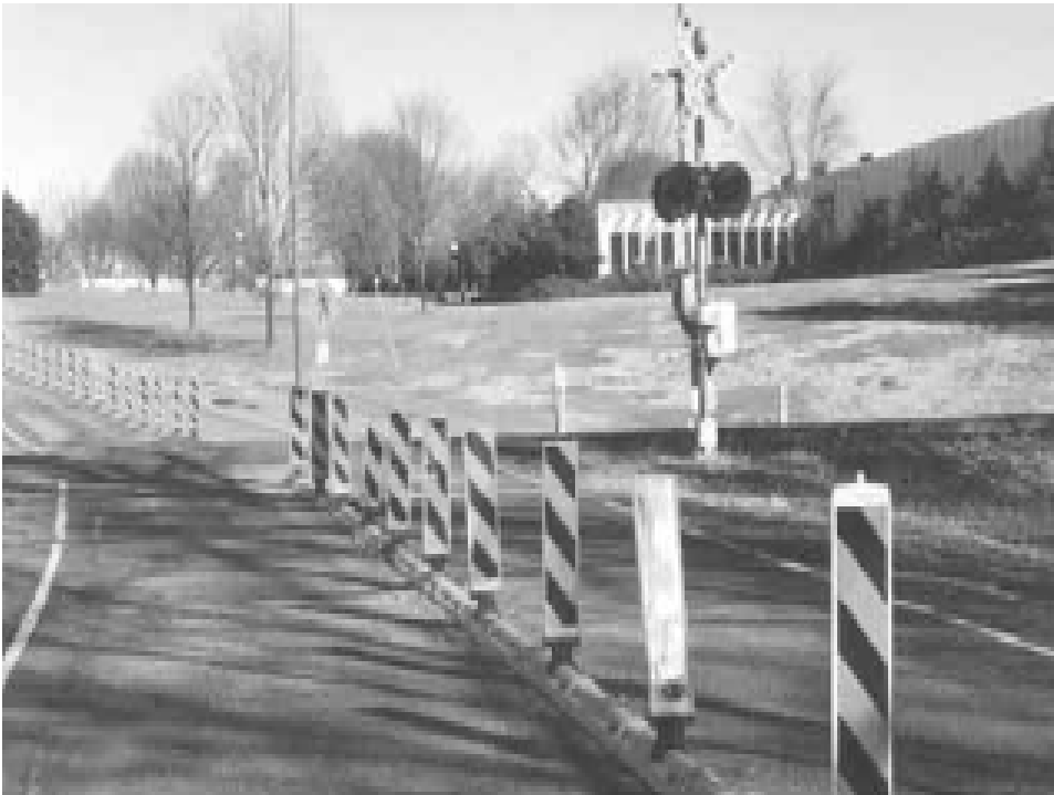
Figure 4: Flexible posts in Harrisburg, North Carolina
