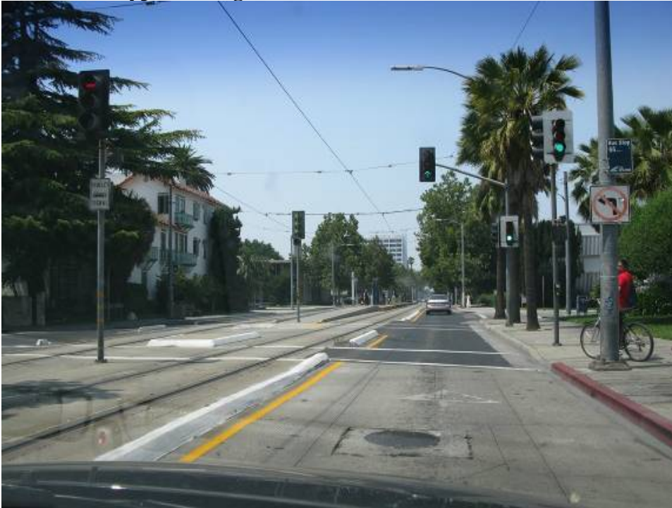
Exhibit 39: Type b.3 Alignment with Barrier Curbs
