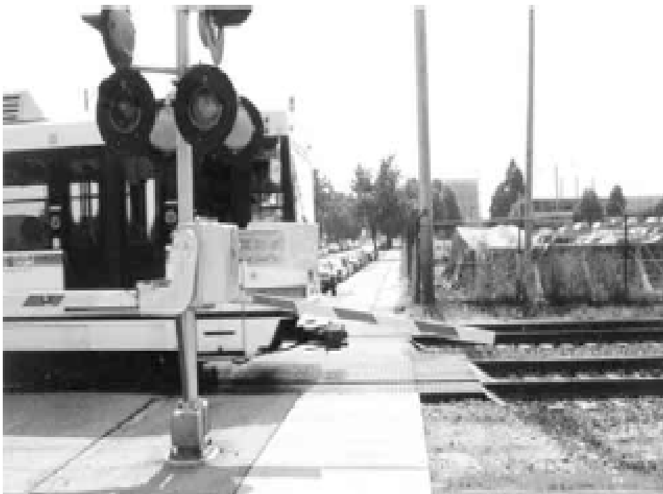
Figure 16: Pedestrian automatic gate
