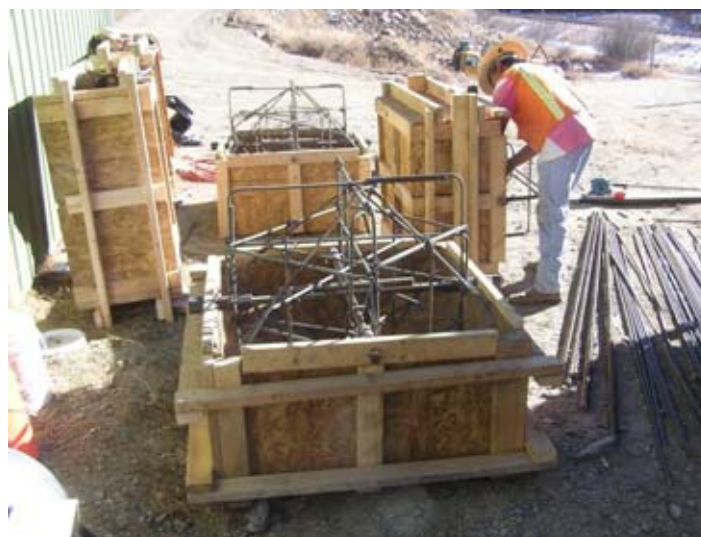
FIGURE 16 Concrete form for cuboctahedrons showing rebar placement.
