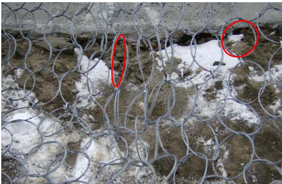
FIGURE 54 Typical deformation of ring-net panel (red outlines compare deformed and unaffected apertures).
