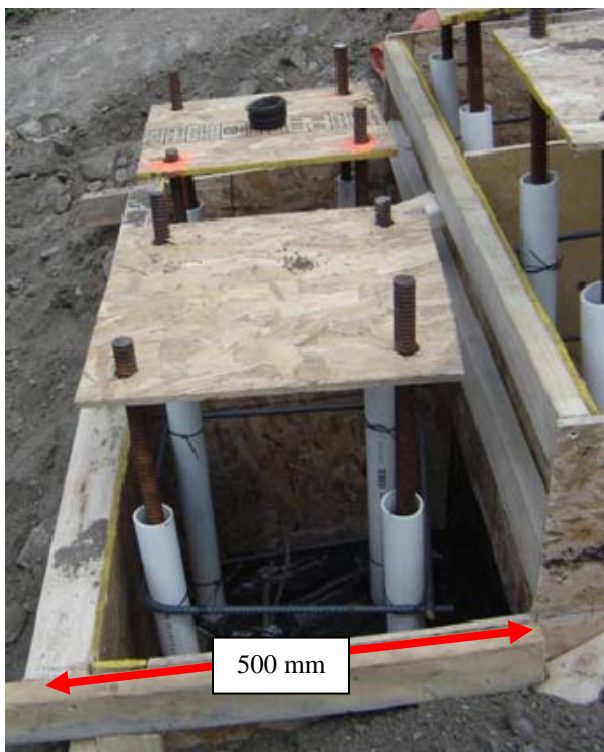
FIGURE 12 Post foundation with concrete forms prior to concrete placement.
