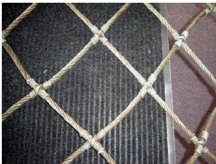
FIGURE 23 Cable net made with 12-mm diameter wire and wire wrap clamp style, diagonal weave.
