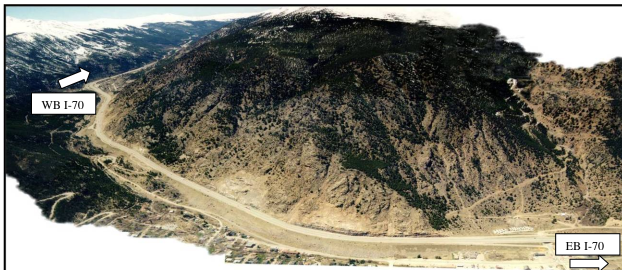
FIGURE 2 Composite photograph of Georgetown Incline.
