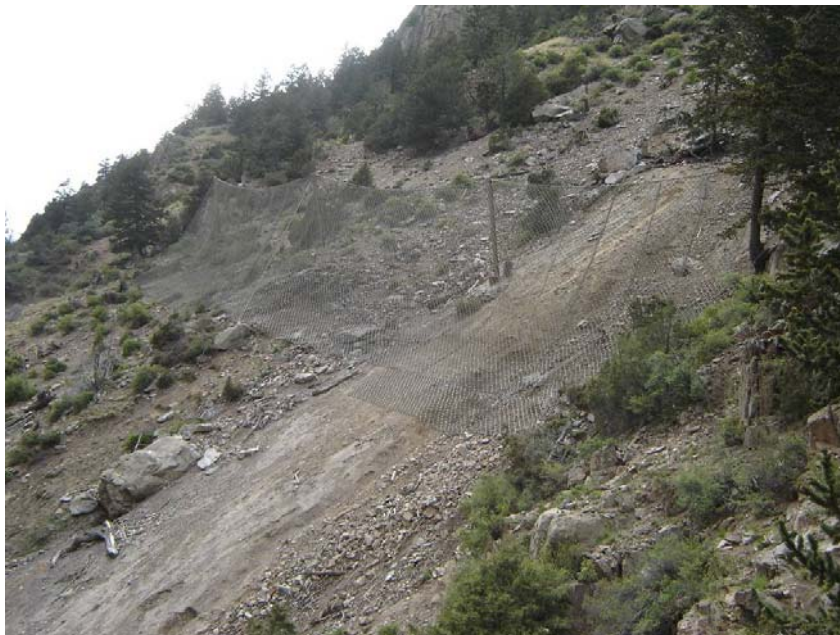
FIGURE 73 View of Attenuator A (looking west).
