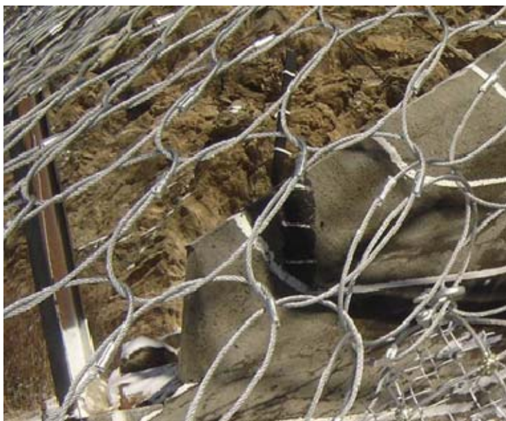
FIGURE 30 Example of cable ring nets.
