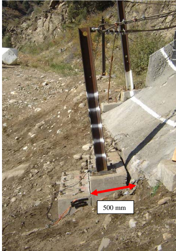
FIGURE 13 Attenuator post attached to foundation prior to testing.
