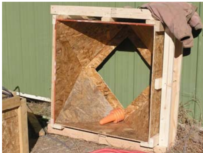
FIGURE 15 Concrete form for cuboctahedrons.
