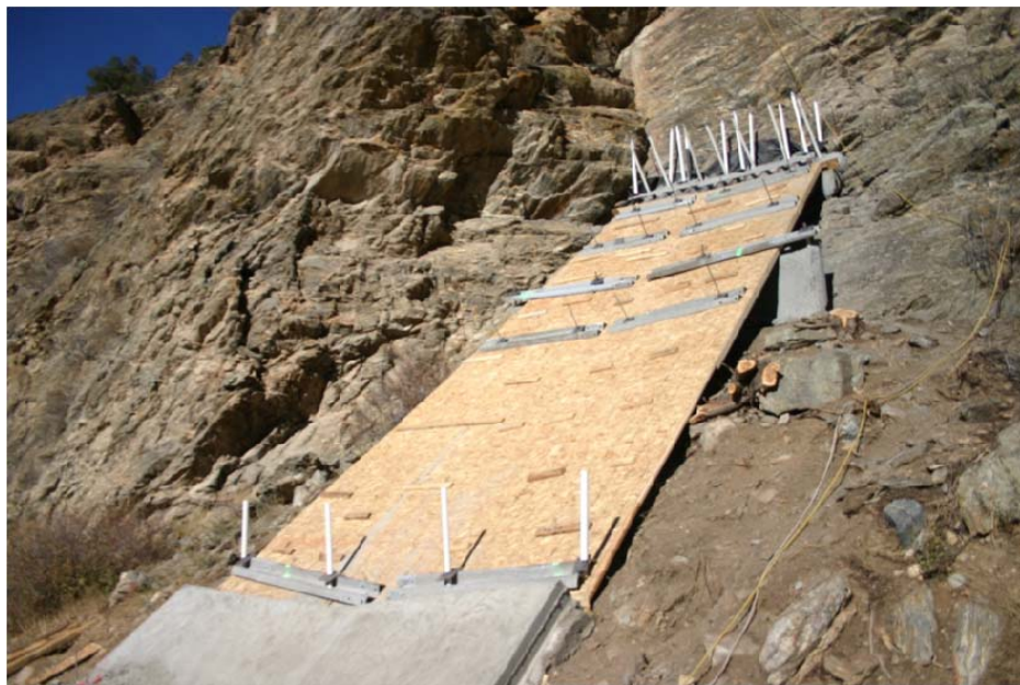
FIGURE 11 Construction of concrete ramp.
