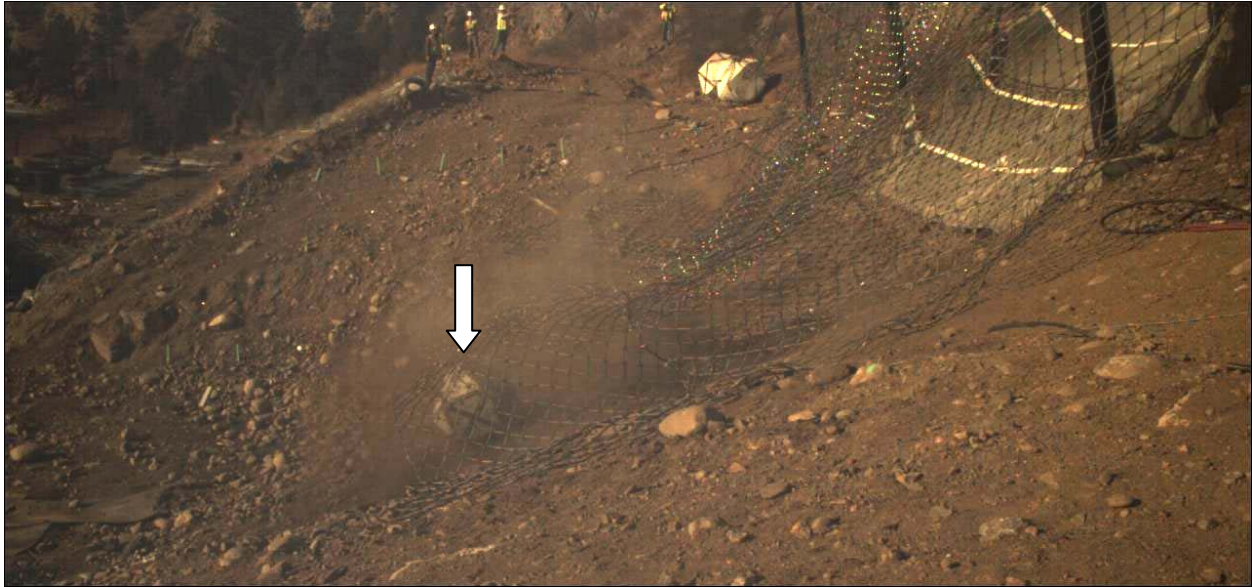
FIGURE 51 Rock released from attenuator with reduced energy.
