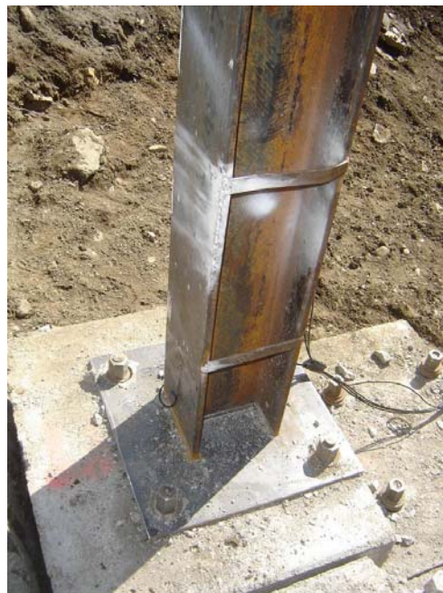
FIGURE 36 Base of fixed post.
