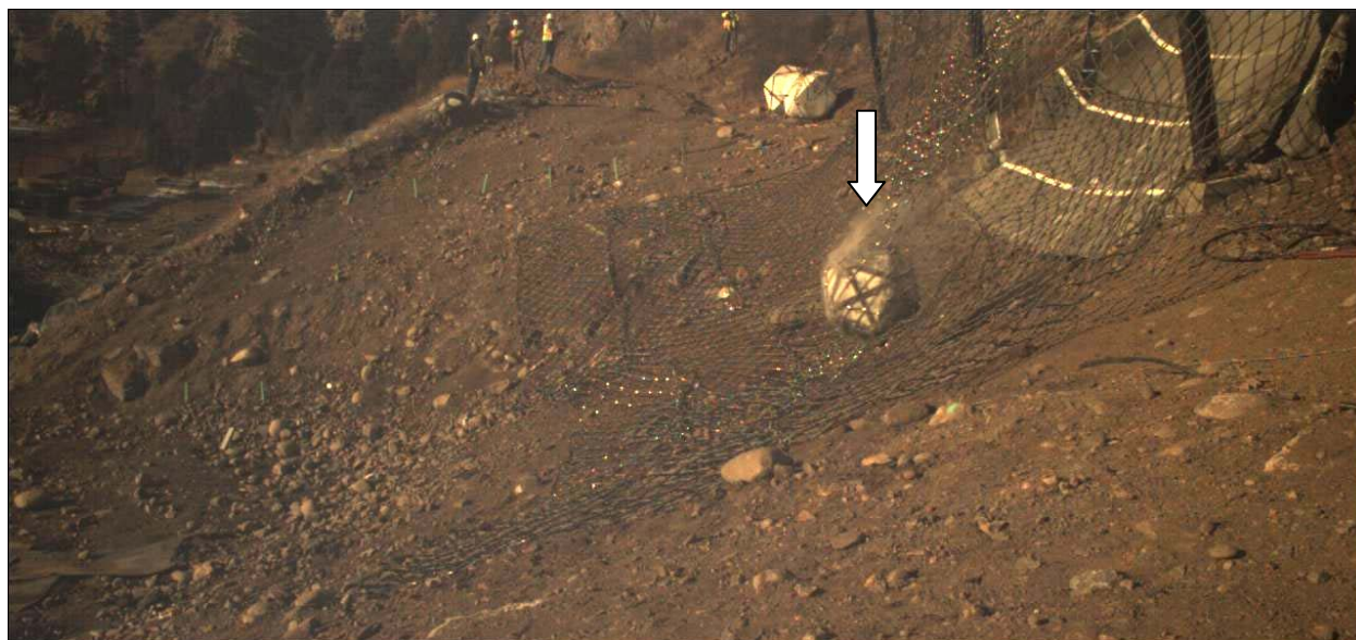
FIGURE 47 Rock traveling into panel.
