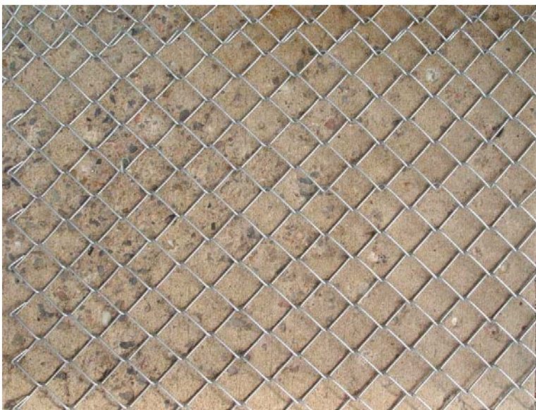
FIGURE 28 Close-up of steel wire (chain link), wire continuous in a horizontal orientation showing how net was hung from support rope on attenuator system (support rope would be at top of photograph).
