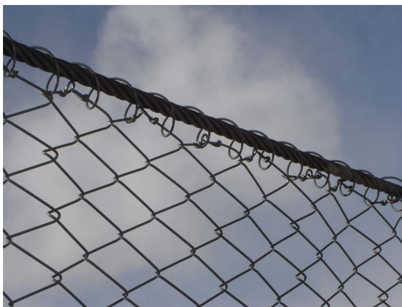
FIGURE 57 Attaching chain-link panel to support cable.
