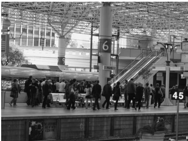
Figure 8 Perth's passenger rail system is completely segregated from freight rail, giving it the ultimate priority.
