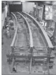
FHWA Curved Girder Bridge FHWC Structures Laboratory
