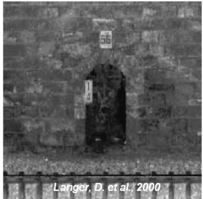
Figure B.1. Image of tunnel niche from laser scanner (40).
