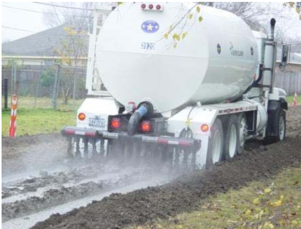
FIGURE 5 Placing cement in slurry form.
