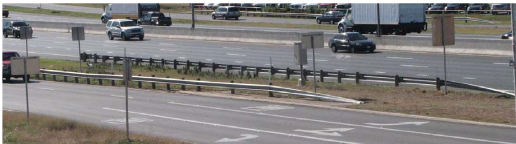
FIGURE 9 Guardrail (350 ft) installed to protect cabinet; move cabinet instead.
