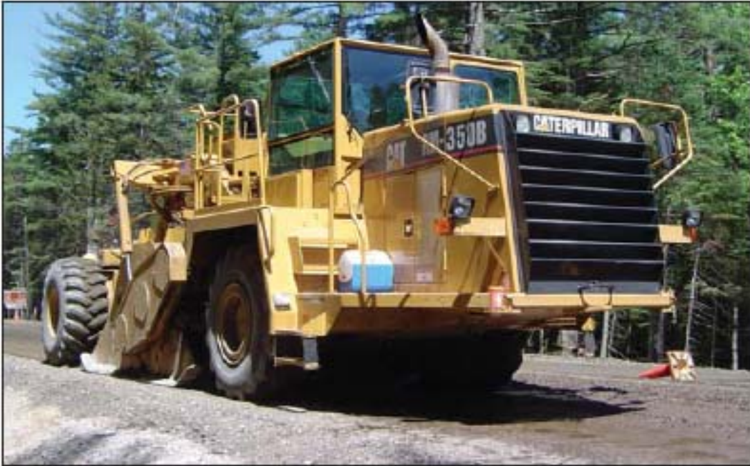
FIGURE 3 Pulverizing a failed asphalt pavement.
