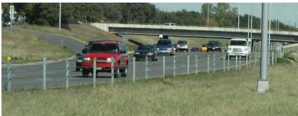
FIGURE 10 Cable barrier adjacent to travel lane receives many nuisance hits.
