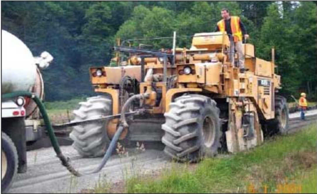
FIGURE 6 Water being injected during mixing operation.
