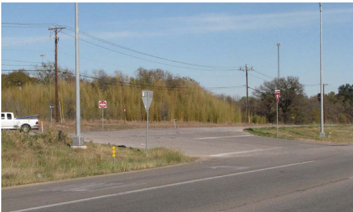
FIGURE 4 Crossover with many unnecessary signs.
