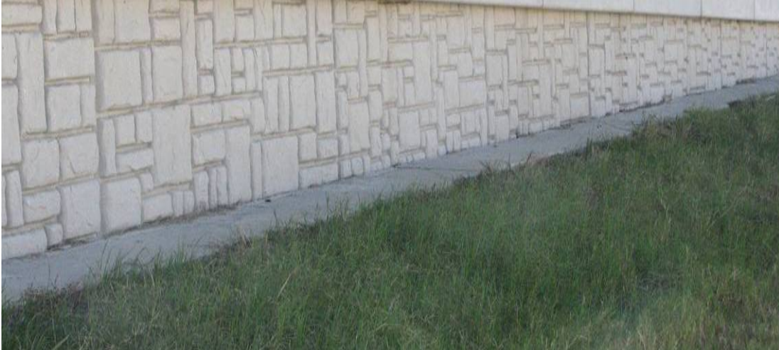
FIGURE 12 Good mow strip along retaining wall eliminates hand trimming.
