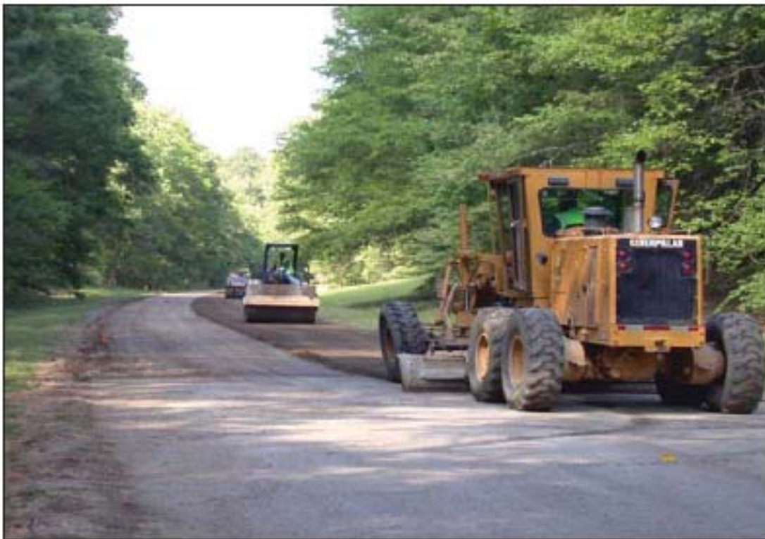
FIGURE 7 Compaction and final grading.
