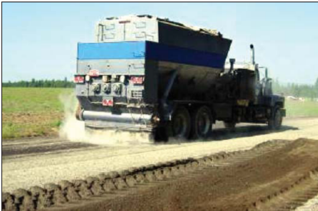
FIGURE 4 Placing cement dry.
