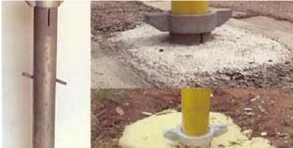
FIGURE 5 Fiberglass sign post with universal mount.
