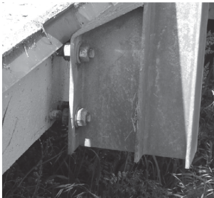
b. Steel barrier
