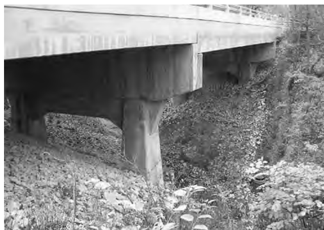
FIGURE 2 Three span box beam bridge over a ravine (Source: Illinois DOT).
