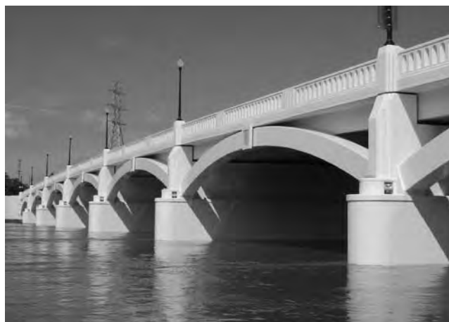
FIGURE 3 Adjacent box beam bridge to replicate an arch bridge (Source: Henry G. Russell).
