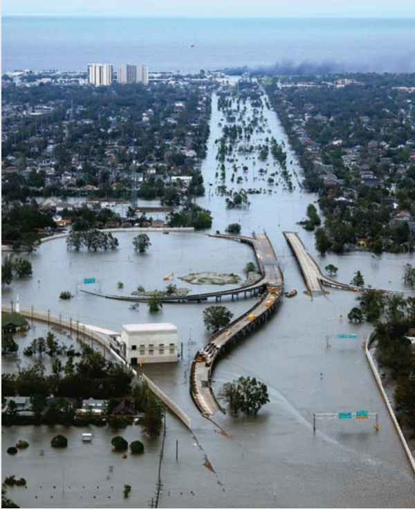
New Orleans, Louisiana, in the aftermath of Hurricane Katrina, showing Interstate 10 at West End Boulevard, looking toward Lake Pontchartrain. This photo is from the U.S. Coast Guard's initial Hurricane Katrina damage assessment overflights of New Orleans. SOURCE: U.S. Coast Guard, Petty Officer 2nd Class Kyle Niemi.
