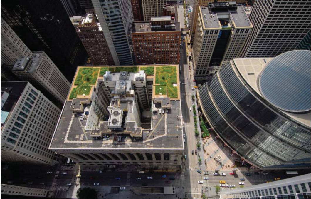
FIGURE 2.3 Green roofs such as this one on Chicago City Hall are aimed at conserving energy. SOURCE: CCAP (2008).
