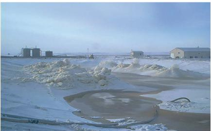
**FIGURE 6.2** Seasonal cycle for freezing, thawing, and evaporation of produced water in Wamsutter, Wyoming. Top: Summer evaporation of melted, relatively pure ice. Bottom: Winter freezing of produced water solution to result in relatively pure water in the form of ice crystals. SOURCE: Used with permission from John Boysen, BC Technologies, Ltd.
