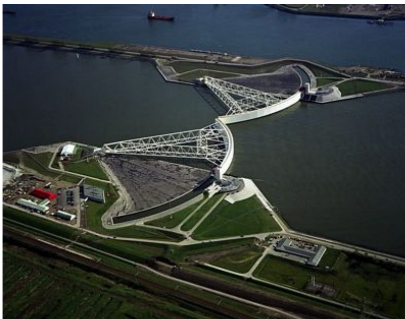
FIGURE 2-5 The Maeslant barrier is a massive flood gate barrier in the Nieuwe Waterweg waterway in the Netherlands. When a storm causes the North Sea to rise, the doors will swing shut (as shown in this image), closing off the river and keeping the water out.
