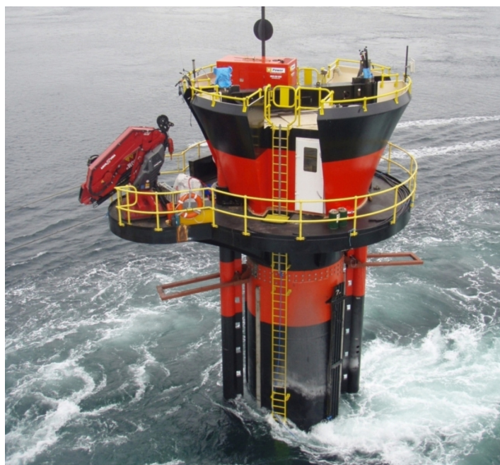
FIGURE 2-7 The world’s first commercial axial turbine tidal stream generator—SeaGen—in Strangford Lough. The strong wake shows the power in the tidal current. SOURCE: Courtesy of Marine Current Turbines Ltd.
