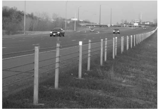
Figure 9 Cable median barrier on a Missouri road.
