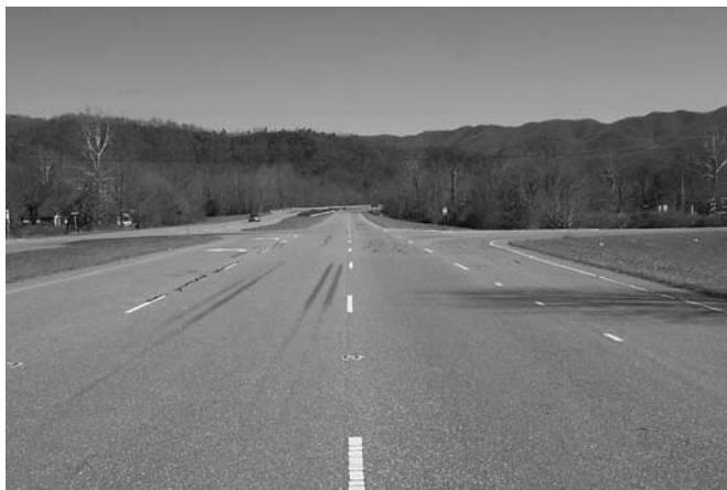
Figure 10 Example of North Carolina road with safety improvements: turn lanes at intersection and improved geometry.
