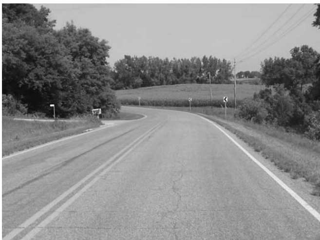
Figure 8 Chevrons enhance curve delineation on a rural Minnesota highway.
