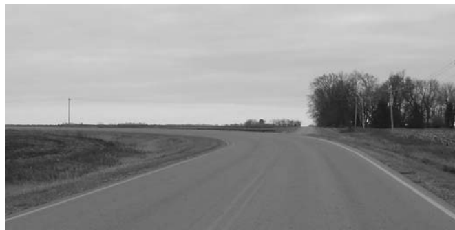
Figure 13 Visual trap at a horizontal curve.
