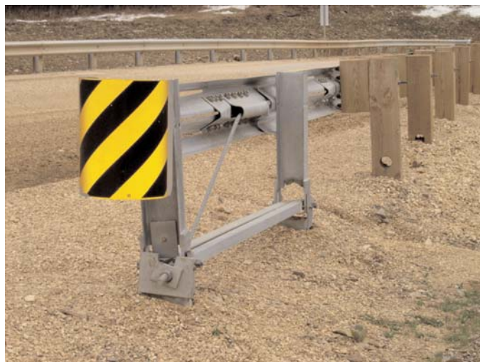
Figure 66. Incorrect stub height (photo: courtesy of South Dakota DOT).
