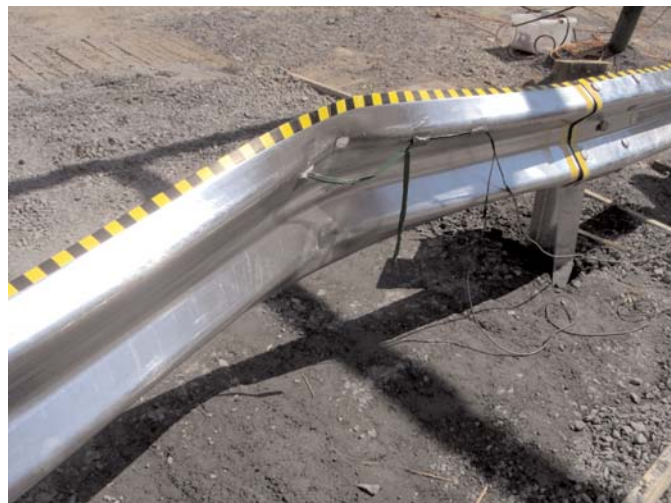
Figure 35. Damage near a hole in Test 07-2.
