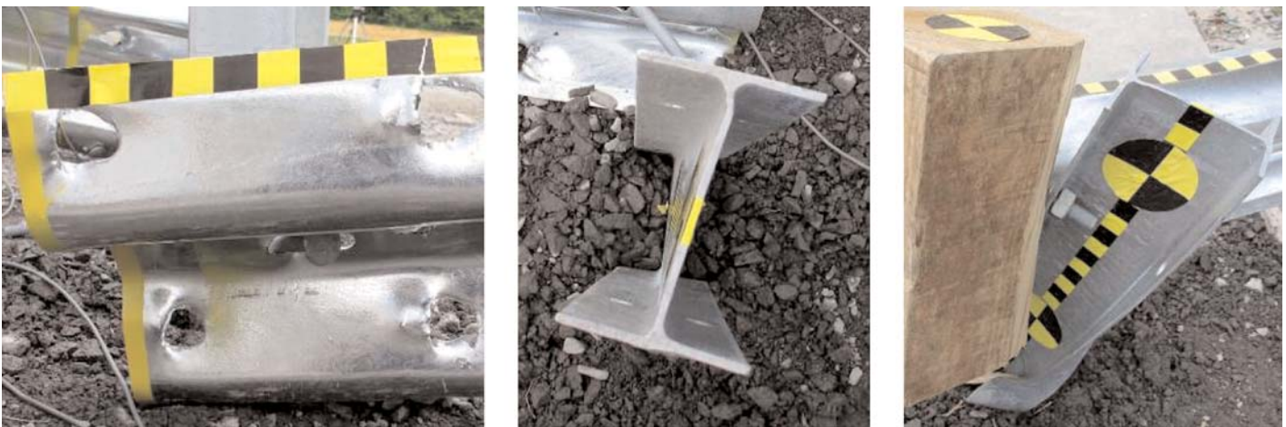
Figure 30. Test 03-7: splice failure (left) and post damage at splice (center) and non-splice location (right).
