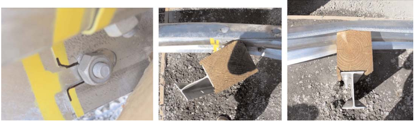
Figure 24. Test 07-4: Detail view of splice bolt damage after test (left) and post damage at splice (center) and non-splice location (right).
