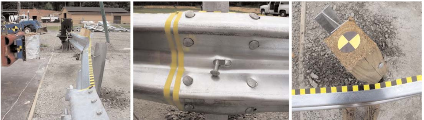
Figure 32. Test 07-5: overall damage (left), detail view of damage at splice (center), and post damage at non-splice location (right).
