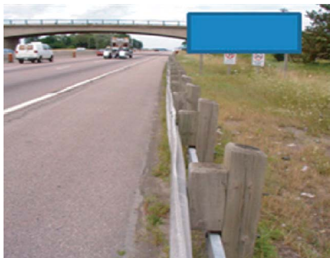
Field Example (courtesy of Ontario Ministry of Transportation)
