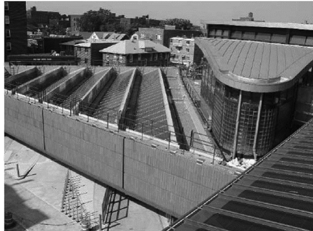
FIGURE 22 Solar roof, Roosevelt Avenue Station, MTA New York City Transit (Source: Greening Mass Transit & Metro Regions: A Synopsis of the Final Report of the Blue Ribbon Commission on Sustainability and the MTA , Metropolitan Transportation Authority, State of New York, Feb. 2009).
