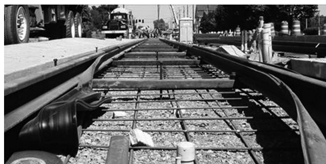
FIGURE 13 Recycled plastic railroad ties used in construction of TriMet’s Interstate MAX Yellow Line.
