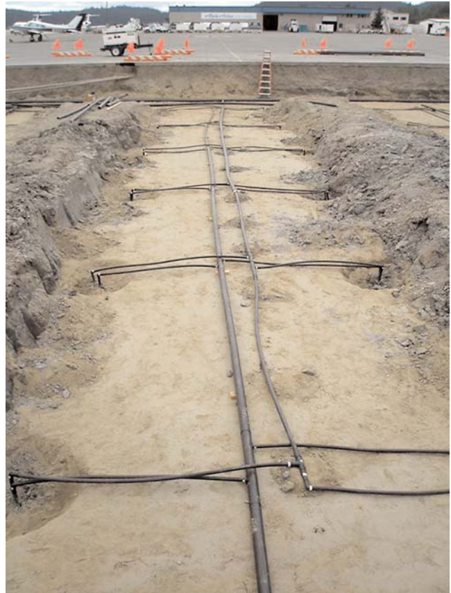
FIGURE 13 Geothermal system installation.
