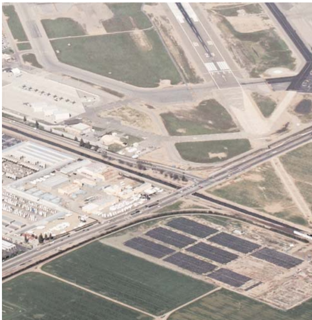
FIGURE 7 Solar photovoltaic array in Fresno, California. The 2.4 mW field shown in the lower right provides more than 50% of the electrical power required for the airport terminal. (Courtesy: Fresno–Yosemite International Airport.)
