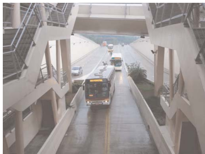
Figure 5 Porto Alegre grade-separated BRT station.
