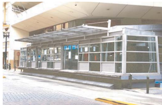
Figure 3 Metrovia downtown BRT station sponsored by private sector.
