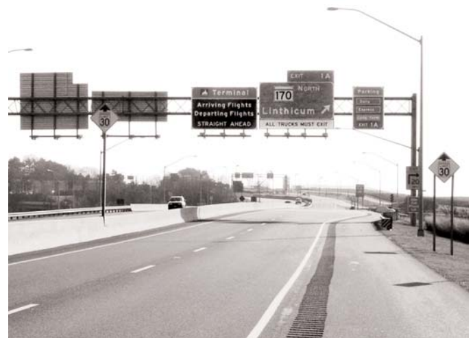
Figure 6-2. Transition from high-speed to low-speed airport roadways at Baltimore/Washington International Thurgood Marshall Airport.
