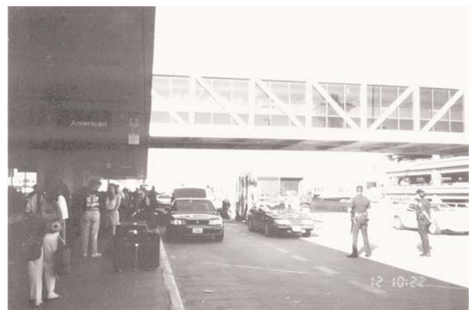
Figure 6-4. Elevated pedestrian bridge at Los Angeles International Airport.
