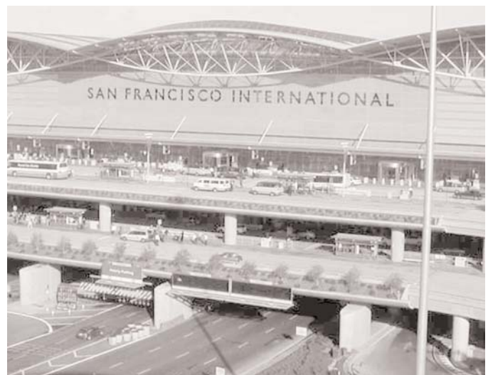
Figure 6-6. Three-level curbside at San Francisco International Airport.
