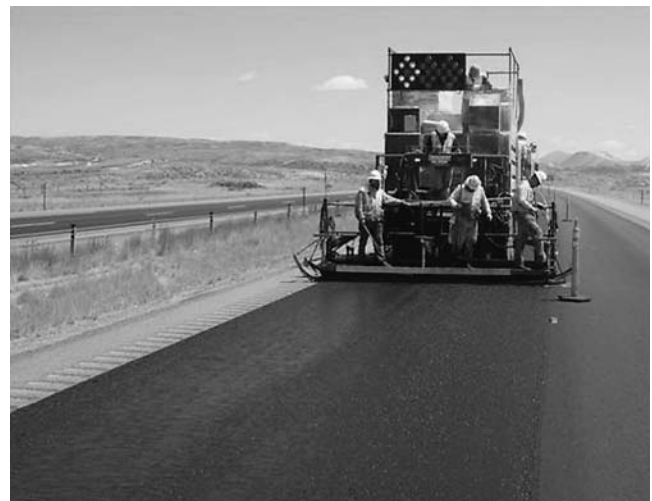
FIGURE 17 Full lane-width microsurfacing (Courtesy: Intermountain Slurry Seal, Inc. 2010).
