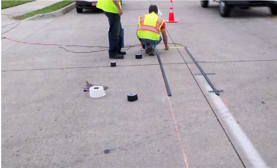
EXHIBIT 4-14 Installing contact closure switches
