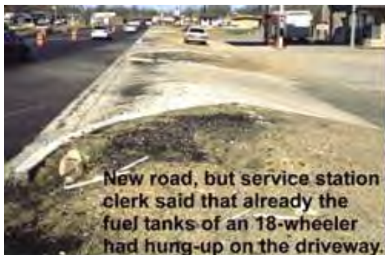
EXHIBIT 3-10 Examples of vertical alignment design problems
