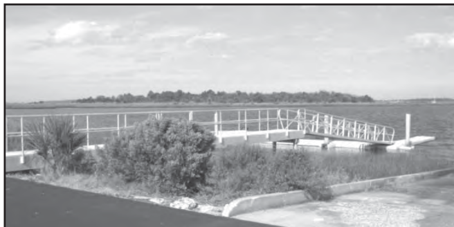
Figure 4. A portion of the constructed seaplane dock at Northeast Florida Regional Airport at St. Augustine (16).
