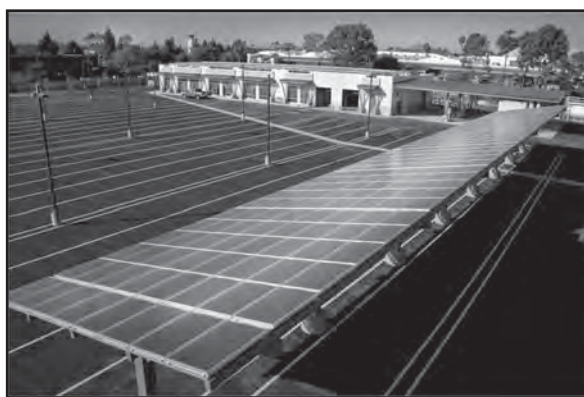
Figure 11. Photovoltaic array at Consolidated Rental Car Facility at Santa Barbara Municipal Airport (Source: Lynn Houston, Santa Barbara Municipal Airport, 2010) (26).
