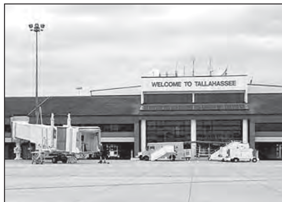
Figure 10. Tallahassee Regional Airport terminal and airfield. (Source: Tallahassee Regional Airport, 2010) (24).
