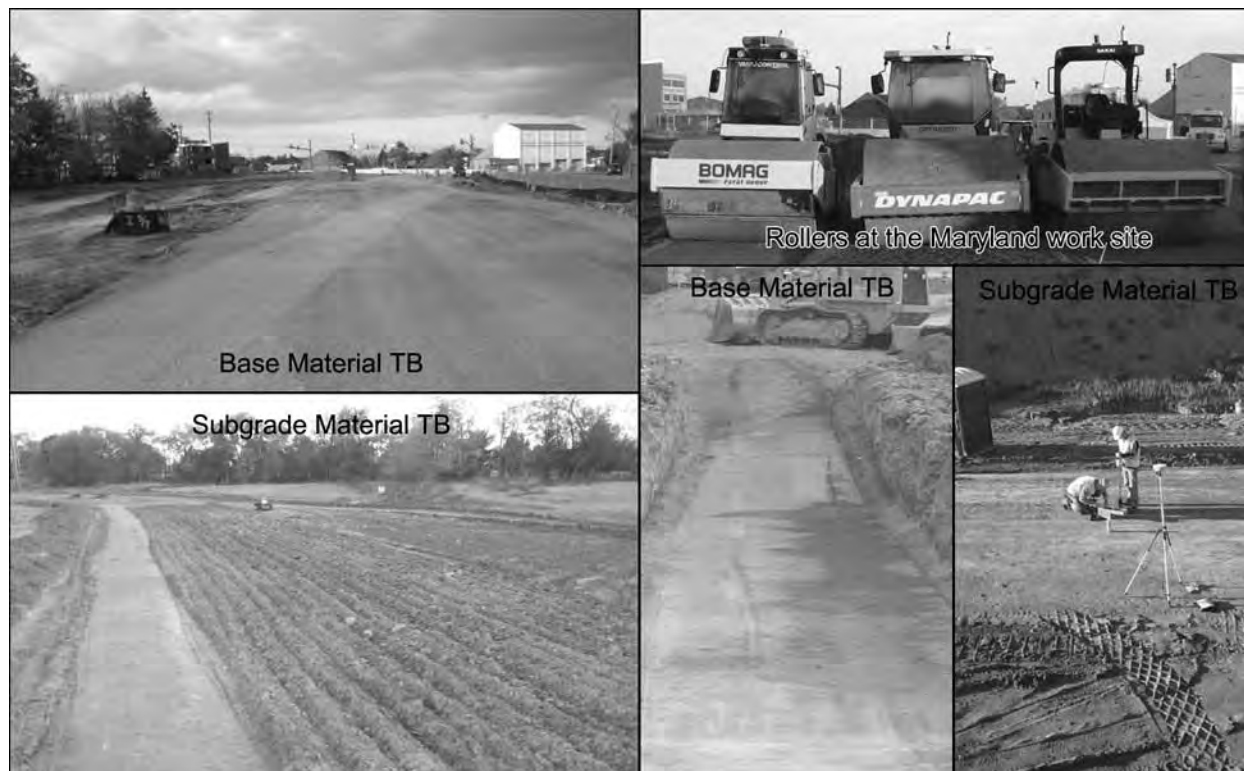
Figure 1.4. IC/CCC rollers and TBs at the Maryland work site.
