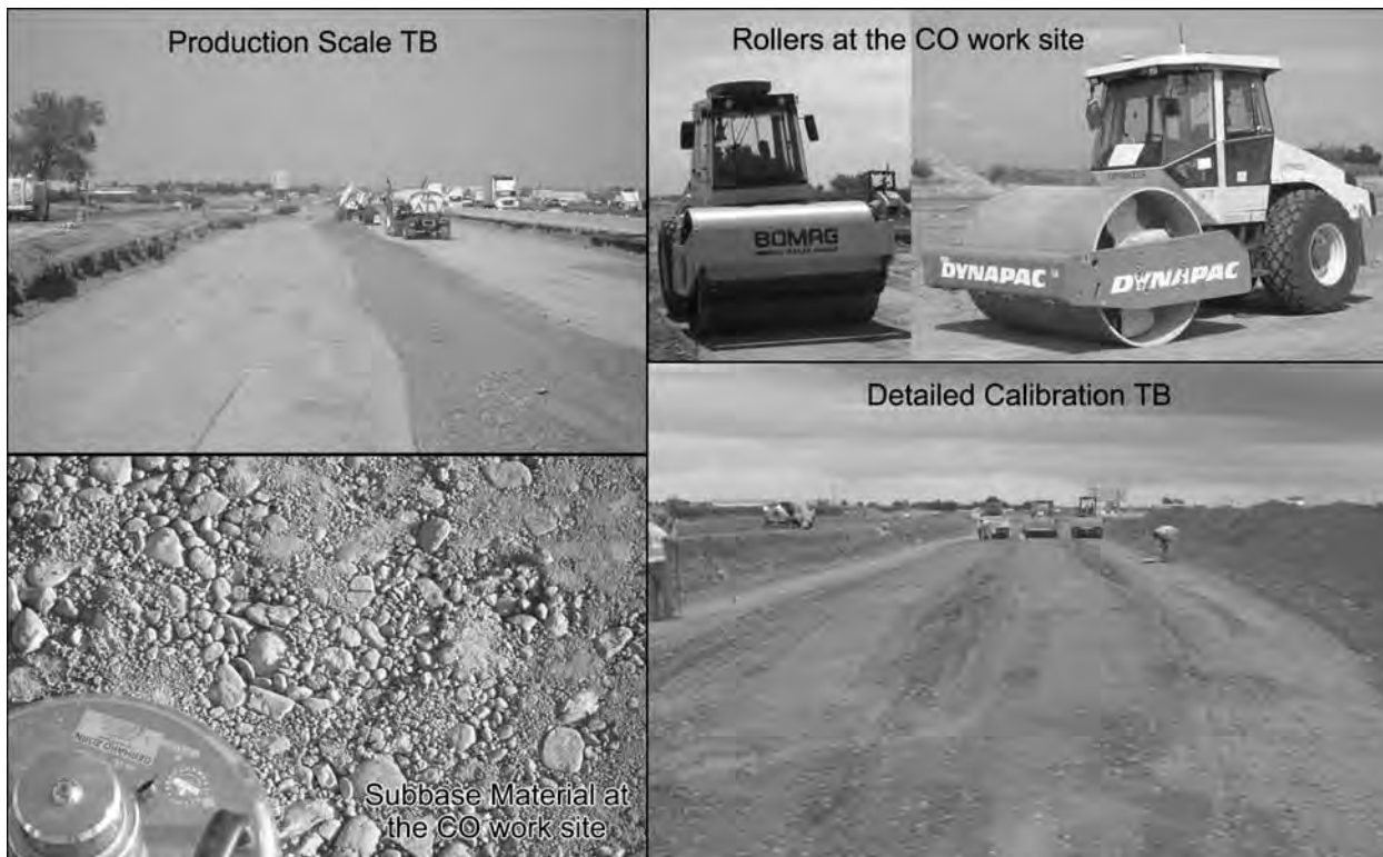
Figure 1.3. IC/CCC rollers and TBs at the Colorado work site.
