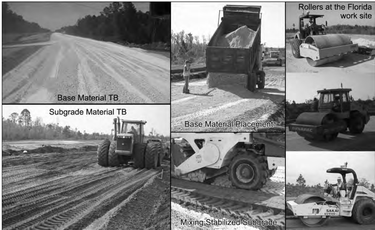
Figure 1.5. IC/CCC rollers and TBs at the Florida work site.
