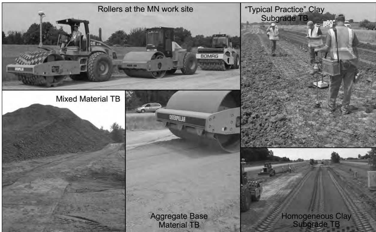
Figure 1.2. IC/CCC rollers and TBs at the Minnesota work site.
