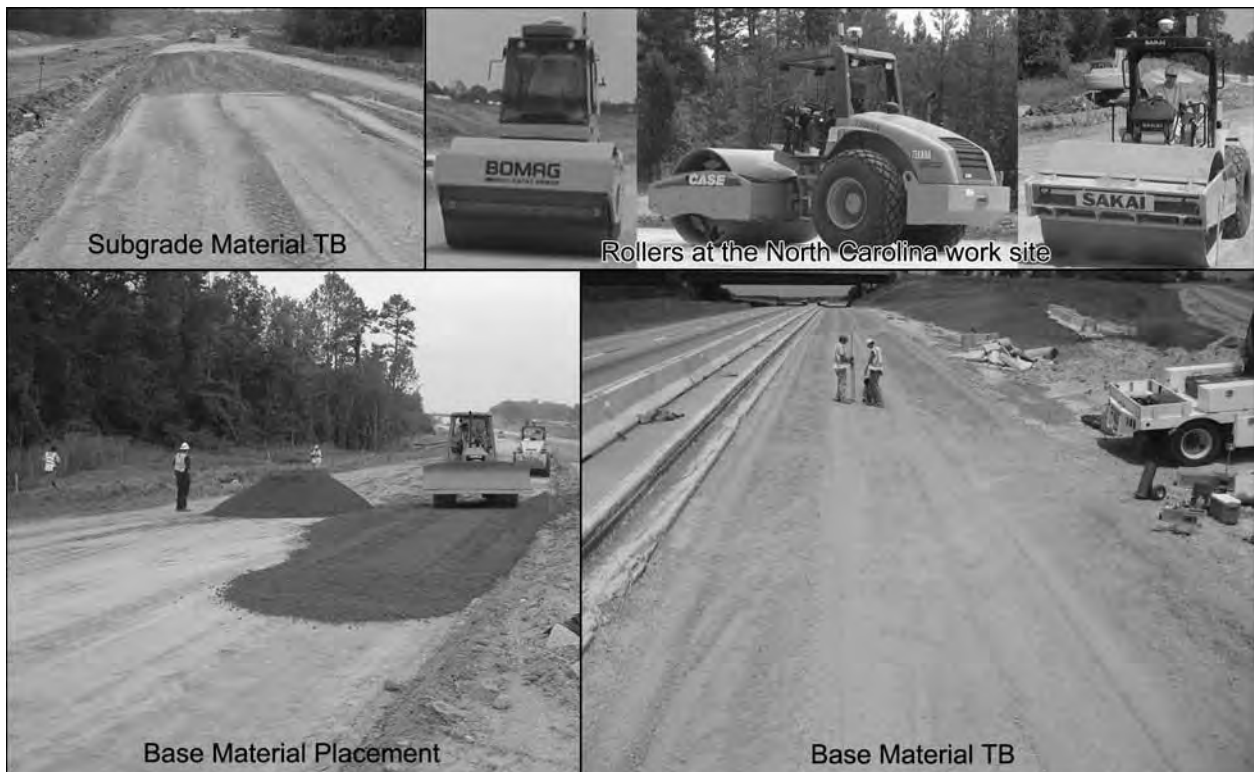
Figure 1.6. IC/CCC rollers and TBs at the North Carolina work site.
