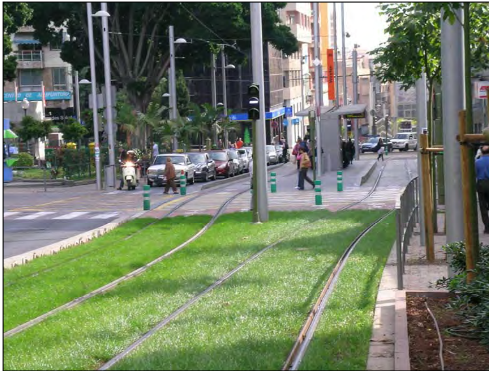
FIGURE 5 Station in which tangent tract is not extended to both sides of the platform, Tenerife light rail.
