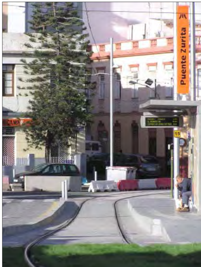
FIGURE 7 Station located in a sag vertical curve, Tenerife light rail (12).
