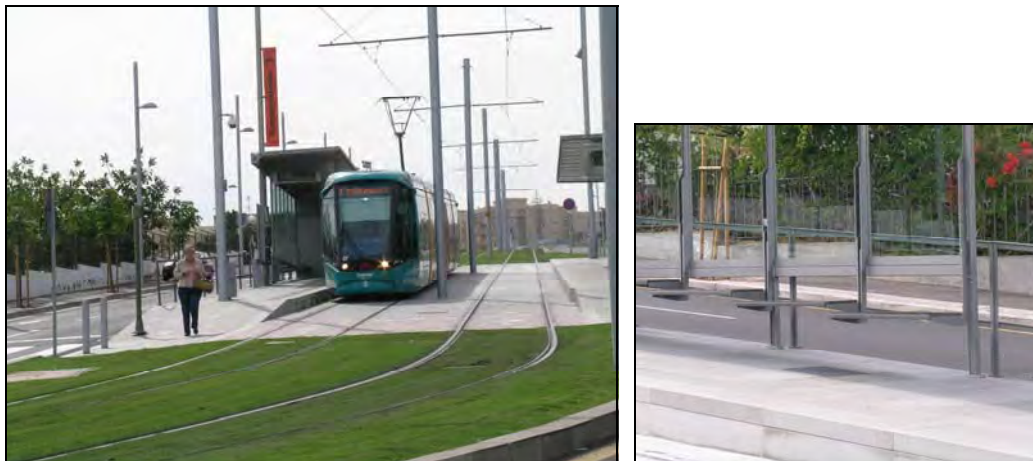
FIGURE 6 Vertical grade of 7.5% at Tenerife light rail station. See the detail of staggered seats in the shelter.
