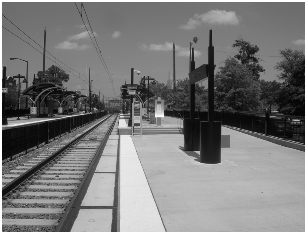
FIGURE 1 Light rail and replica trolleys have separate but adjacent platforms in Charlotte. The trolley boarding area is at the front of the above picture, and the raised light rail platform is in the rear.
