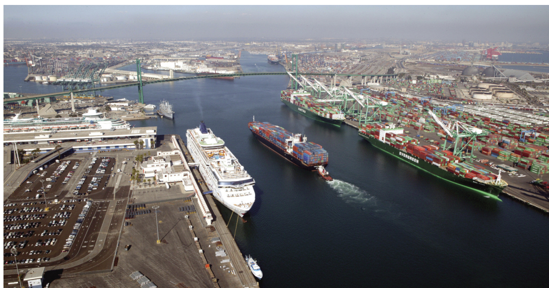
PHOTO: PORT OF LOS ANGELES
