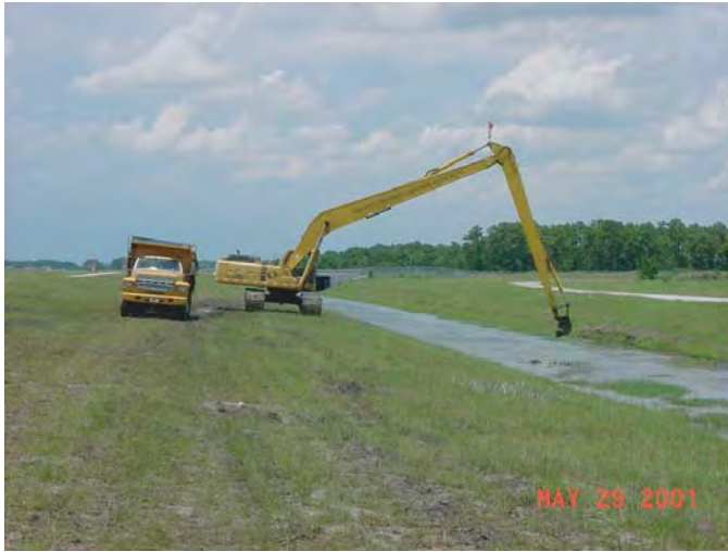
Maintaining drainage ditches improves water flow and reduces food and cover sources for birds. (Photo E. Cleary)
