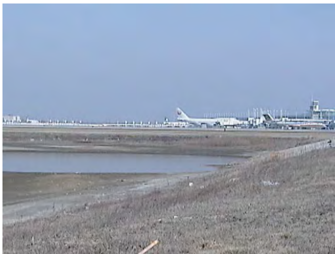
This is the storm water detention pond shown in the previous photo, almost completely drained following an early spring rainstorm. (Photo courtesy USDA)
