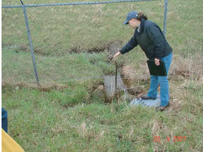
Properly installed and maintained fencing will keep most large mammals out of an airport. Places where drains run under the fence should have guards installed to prevent animals from crawling under the fence. (Photo E. Cleary)
