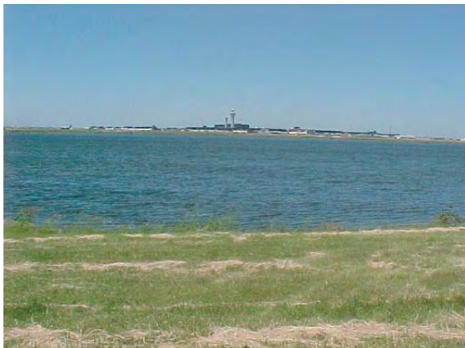
Storm water detention basins should be designed to drain completely within 48 hours following the design storm. See next photo. (Photo courtesy USDA)
