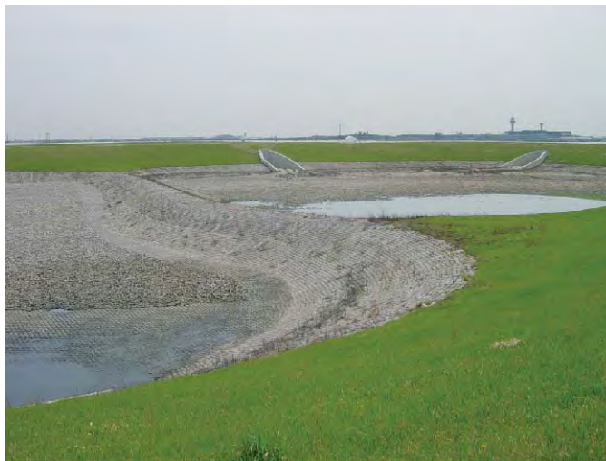
Even though this detention pond was originally designed to drain within 48 hours following the design storm, additional work is needed to ensure it drains completely. (Photo courtesy FAA)
