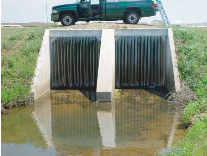
Plastic strips were hung over this drain to stop swallows from nesting in it. (Photo P. Robinson)
