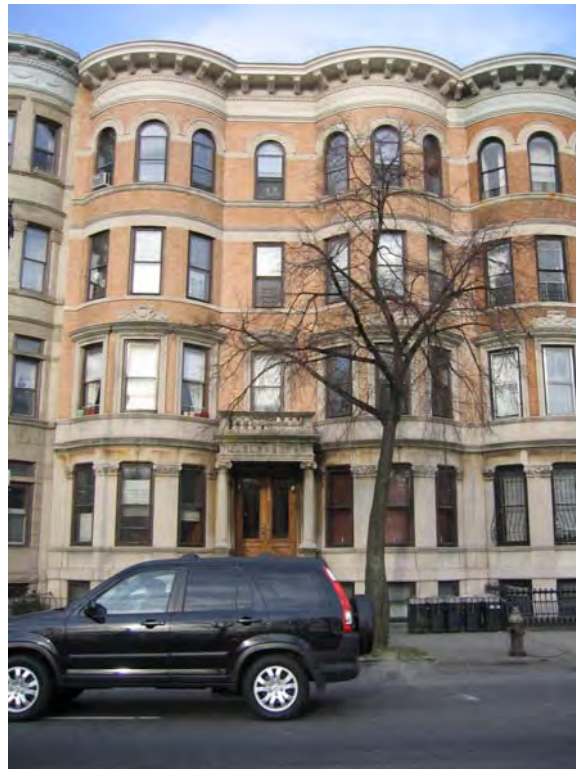
Figure A-5: New York Typical Residential Construction
