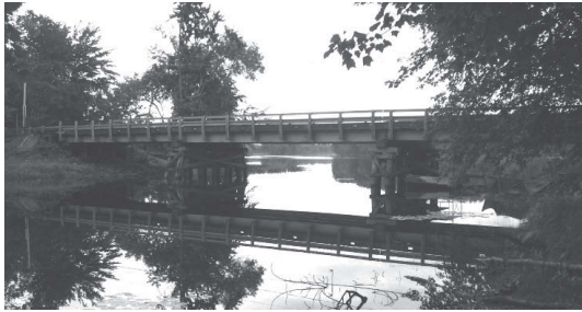
An aging bridge in Old Town, Maine, was replaced with three precast spans, saving months from the schedule required for cast-in-place concrete construction.
