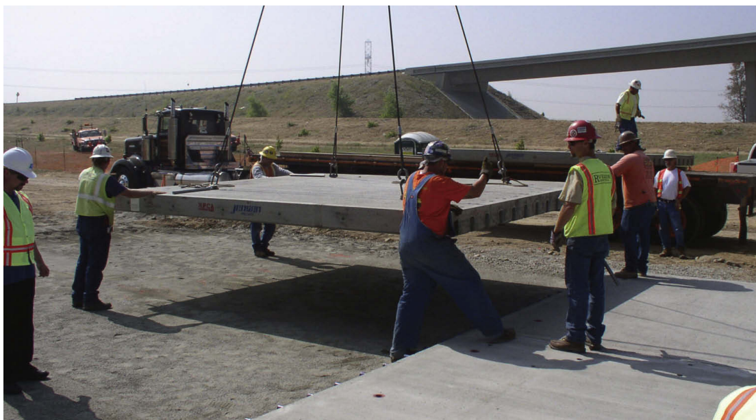
PHOTO: DYNATEST CONSULTING INC.
